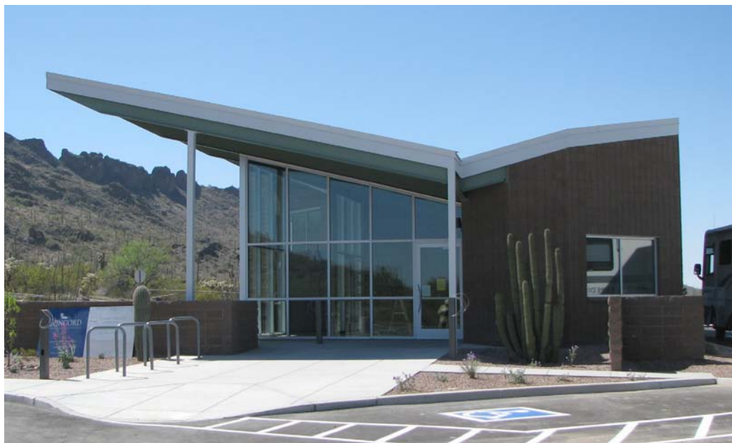
The new Visitor Center at Picacho Peak State Park has been completed. The building has been submitted for review to the U.S. Green Building Council; its certification as Gold in Leadership in Energy and Environmental Design (LEED) is pending.
