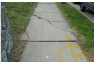
Sidewalk in Condition Rating 4
