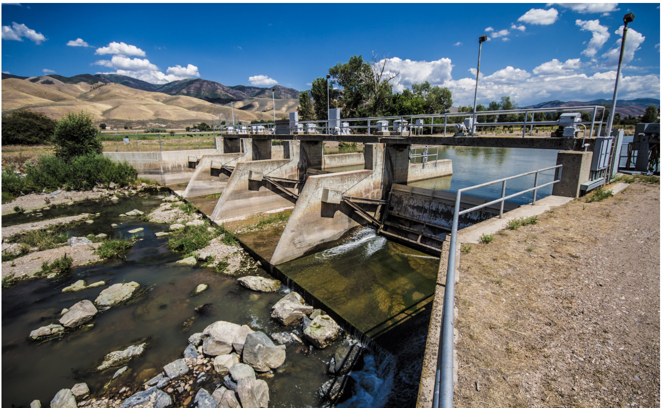
Fig 2.2: Dewatering downstream of the Stoddard Diversion.
