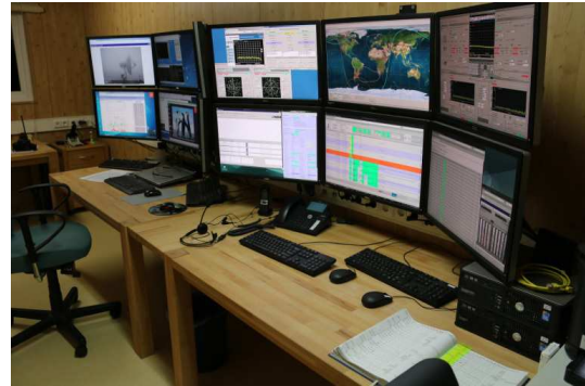
Fig. 3 The new control room with the operator desk for VLBI work of the BKG and satellite tracking of the DLR.
