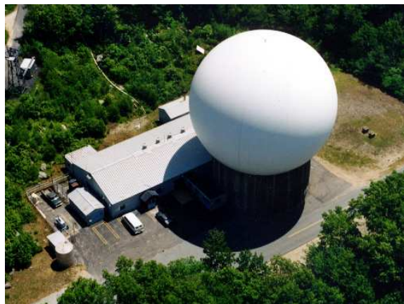
Fig. 1 Aerial view of the radome and facilities of the Westford antenna. (For scale the diameter of the radome is 28 m.)
