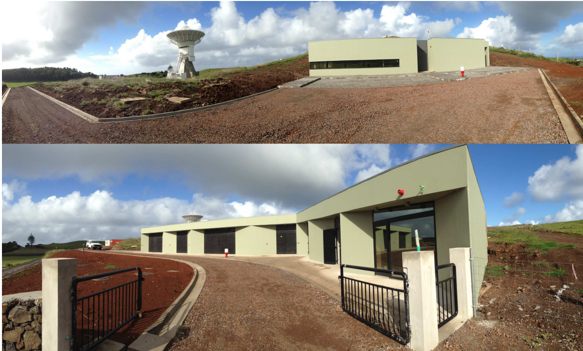
Fig. 2 Status of construction of the control building at the RAEGE station in Santa María (Azores).
