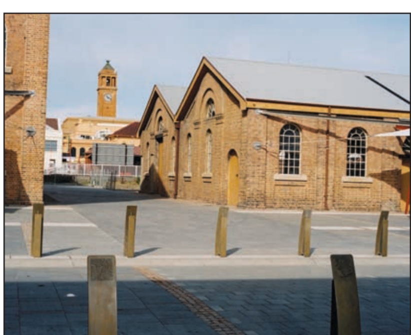
View between the Locomotive Boiler Shop and Blacksmith's & Wheel Shop (SOURCE: HDC 1997)
