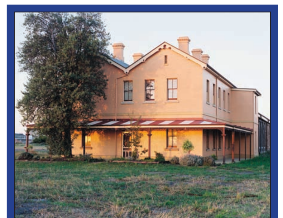
F Divisional Engineer's Office c1883 (SOURCE: HDC 1997)
