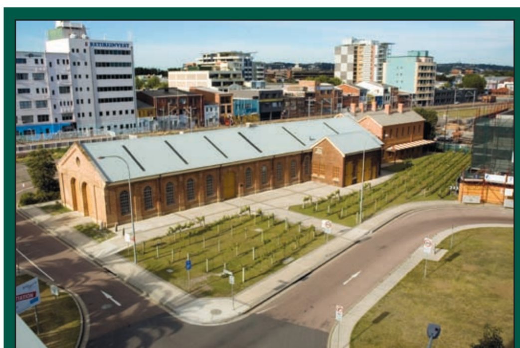
E Locomotive Machine Shop c1874 (SOURCE: HDC 2005)
