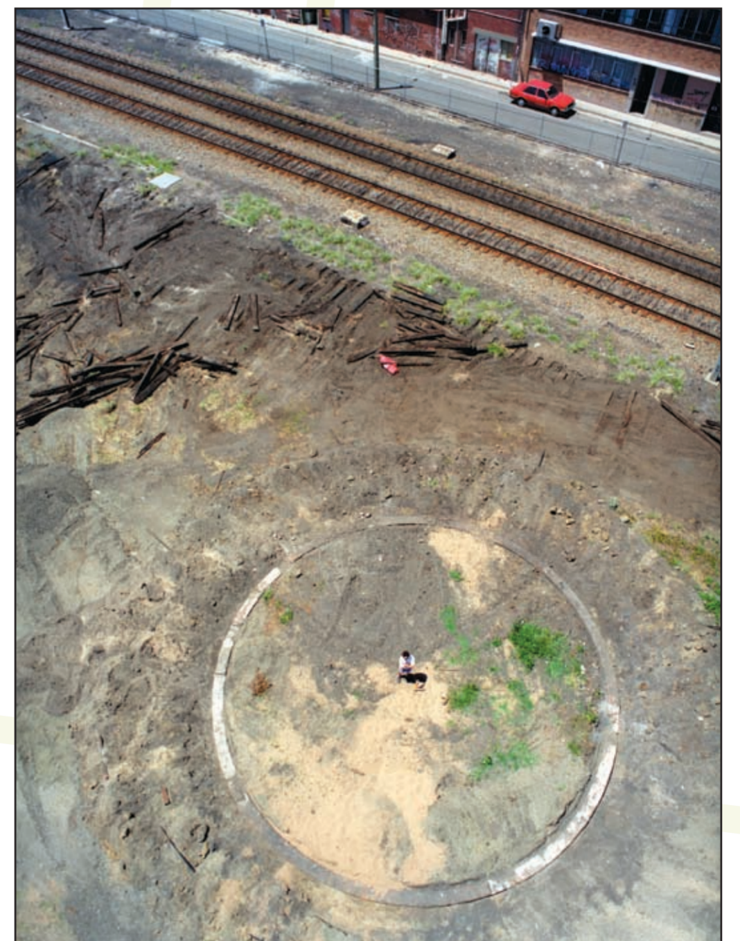
The Turntable during excavation works in 1994 (SOURCE: HDC)
