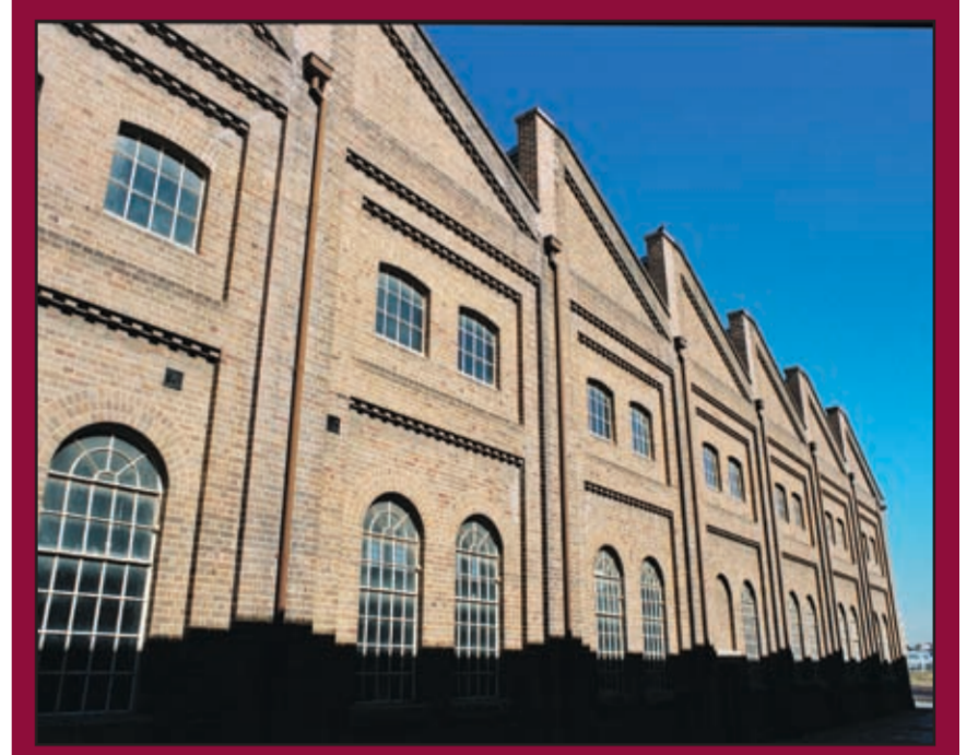
C Saw tooth roof profile of the New Erecting Shop (SOURCE: HDC 1997)
