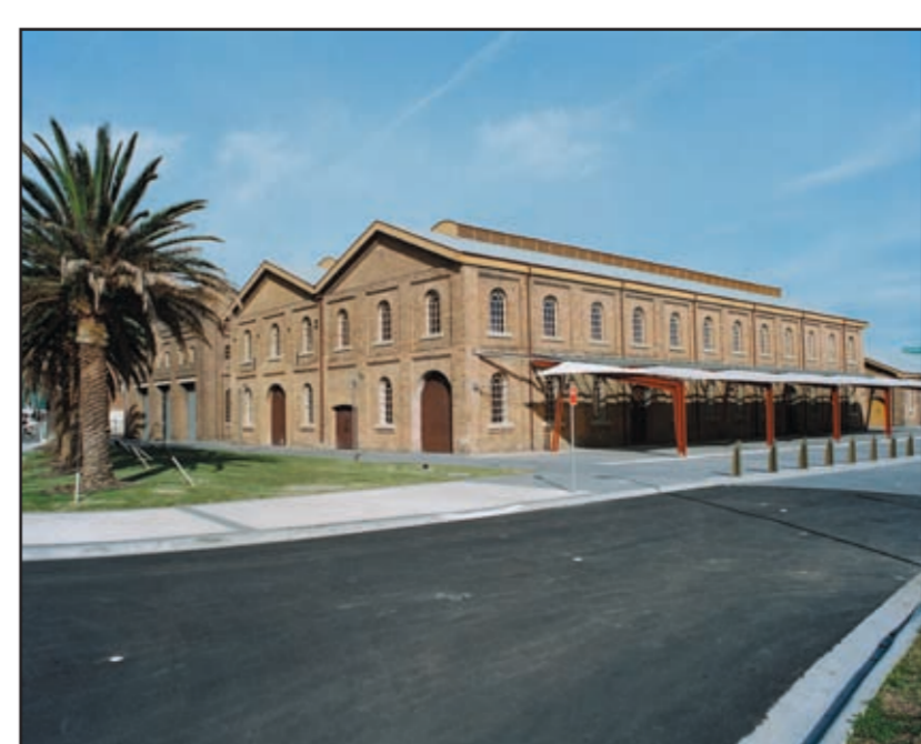
The Locomotive Boiler Shop c1887 (SOURCE: HDC 1997)
