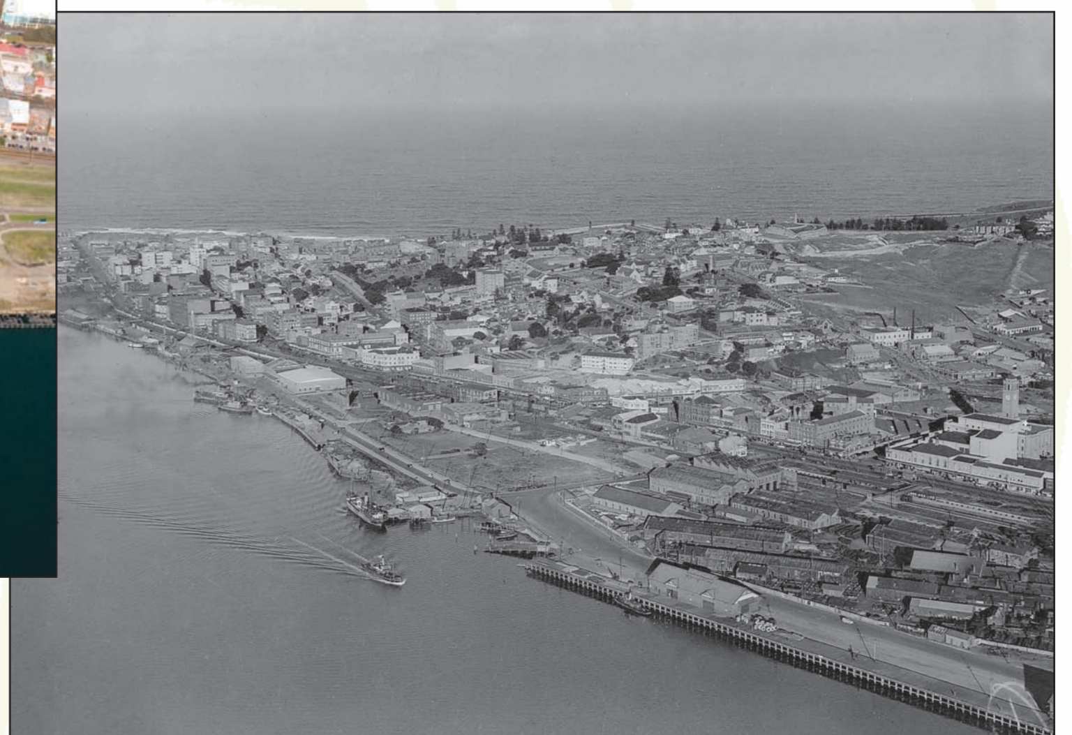
Lee Wharf and Railway workshops circa late 1930s (SOURCE: STATE RECORDS NSW)
