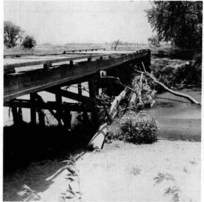
Water flowing at high velocities is capable of causing erosion to streambanks and fill around bridge abutments as well as transporting large objects.
