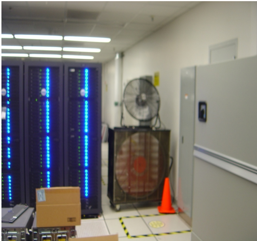
Fans were used to redirect air
