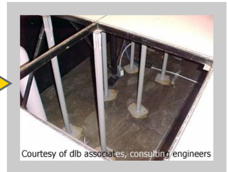
Empty Floor & Ceiling Cavities
