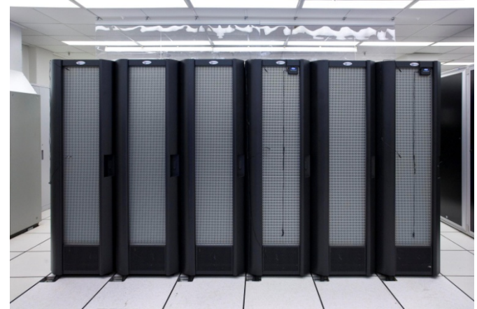
Rear Doors (closed)
