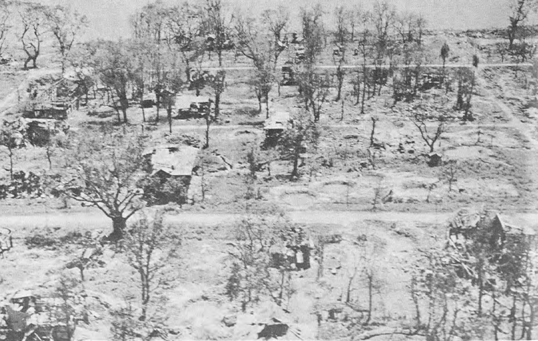
BOMB DAMAGE AT MYITKYINA
