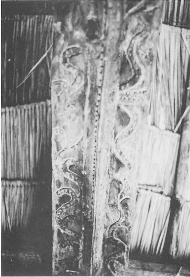
Figure 86. B. Chāngm̄ Luang: The northern girder in the eastern part of the nyoe' nyū seen from below, showing scrolls partly broken through.
