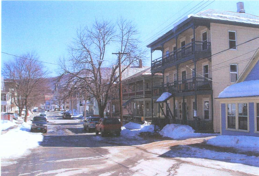
9. View looking east down Williams St. Ext. # 64, 66, 68 in right half of photo.
