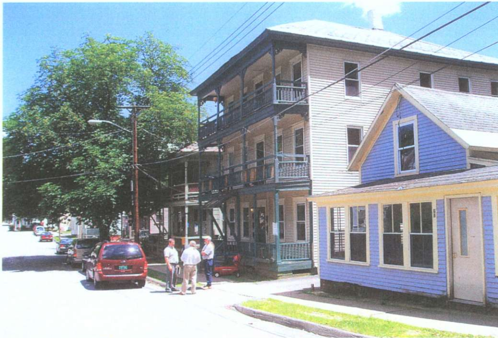
19. View of 66 Williams Street top (center) and bottom.
