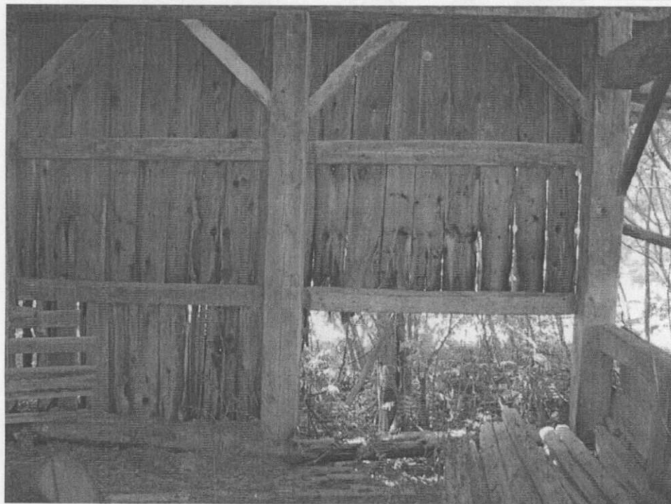
Picture 8. Interior South Wall.
