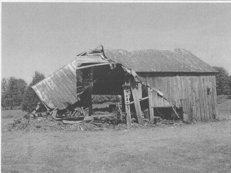
Picture 4. Exterior South Wall.
