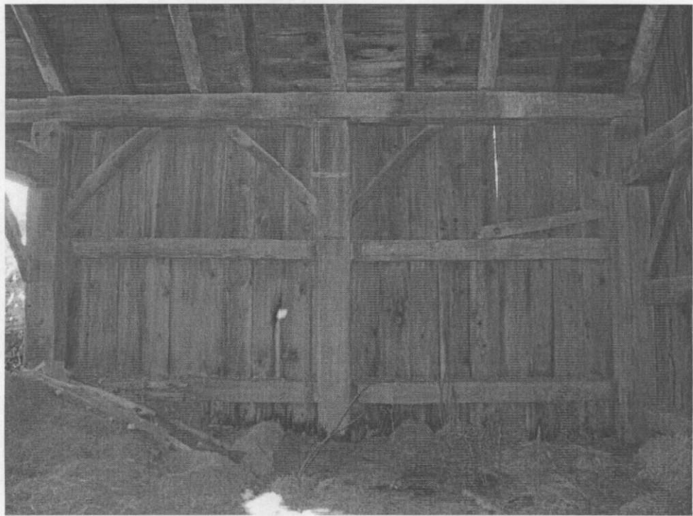
Picture 6. Interior North Wall.
