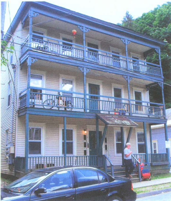
20. Front elevation of 66 Williams St. Ext.
