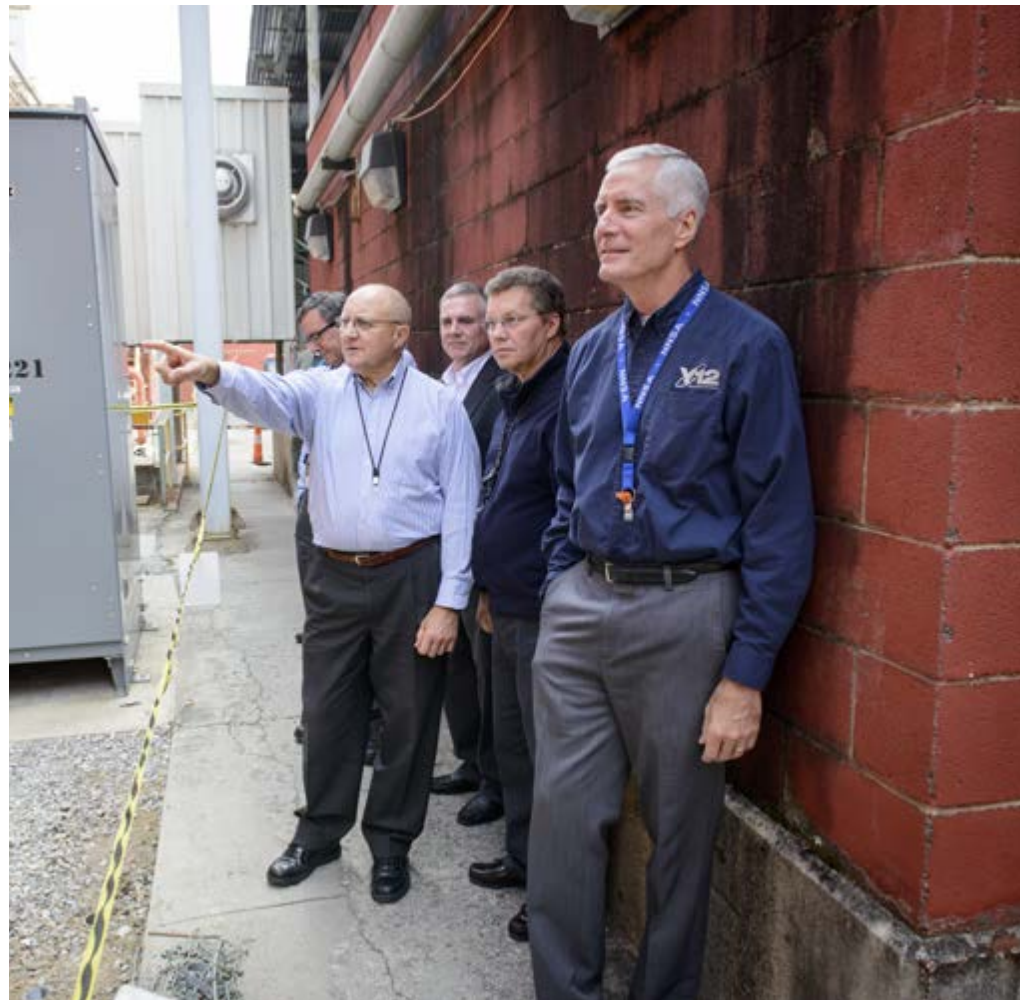
The Y-12 team shows NNSA Uranium Program Manager Tim Driscoll, front, infrastructure upgrades during a tour of Building 9995.
