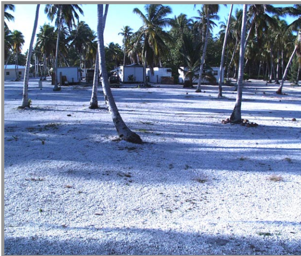
Lack of coral fill between newly constructed garages and original resettlement camp.
