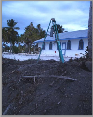
Mounds of dark soil/fill placed on the beach adjacent church.
