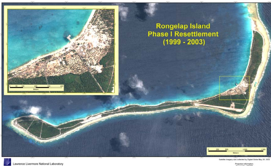
Figure 3. Satellite image of Rongelap Island showing (insert) the location of the community center where surface soil was removed and replaced with clean crushed coral fill (approximately 11.4 ha or 36.1 acres).
