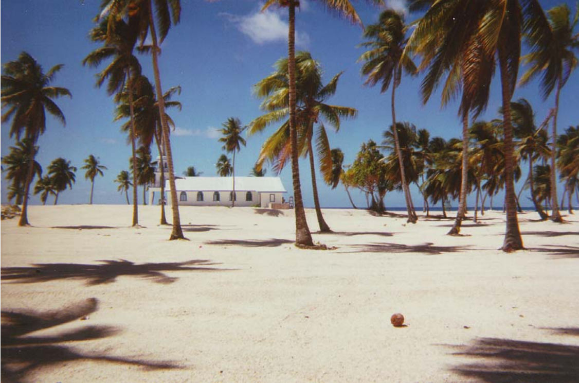
Figure 4. View of the village area on Rongelap Island after the addition of crushed coral fill. The refurbished church in the background is the only original building remaining on the island from 1985.
