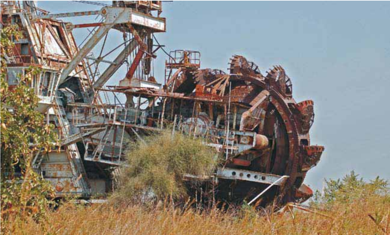
The rusting wreckage of the Jonglei canal excavator lies in the unfinished main channel. This failed venture illustrates the risks associated with developing large-scale projects in socially and environmentally sensitive areas without local support
