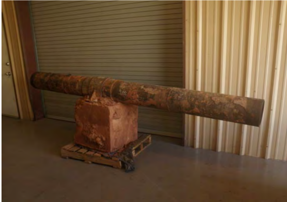
Photo 6 – Segment removed for metallurgical testing
