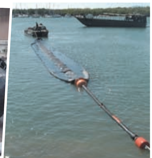
The TFBS in the water being positioned for anchoring
