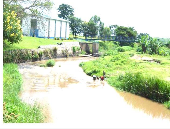
Soil erosion leads to turbid water in the River Manafwa. This is near the water abstraction point of water treatment works of National Water and Sewerage Corporation in Mbale
