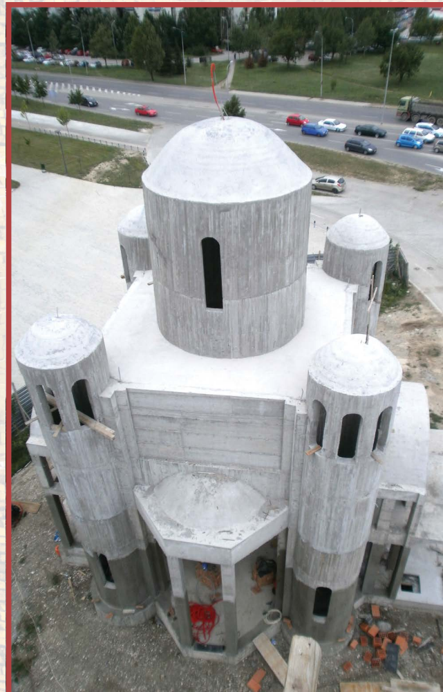
Црква – градба Church – Construction
