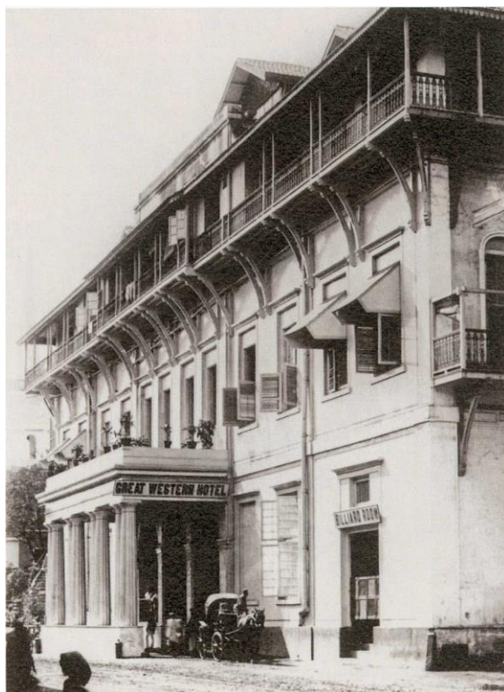
FIGURE 3.4 & 3.5. (Above) The Byculla Hotel and (below) the Great Western Hotel, Fort. Notice the entrance to the Billiard Room on the ground floor of the Great Western.
