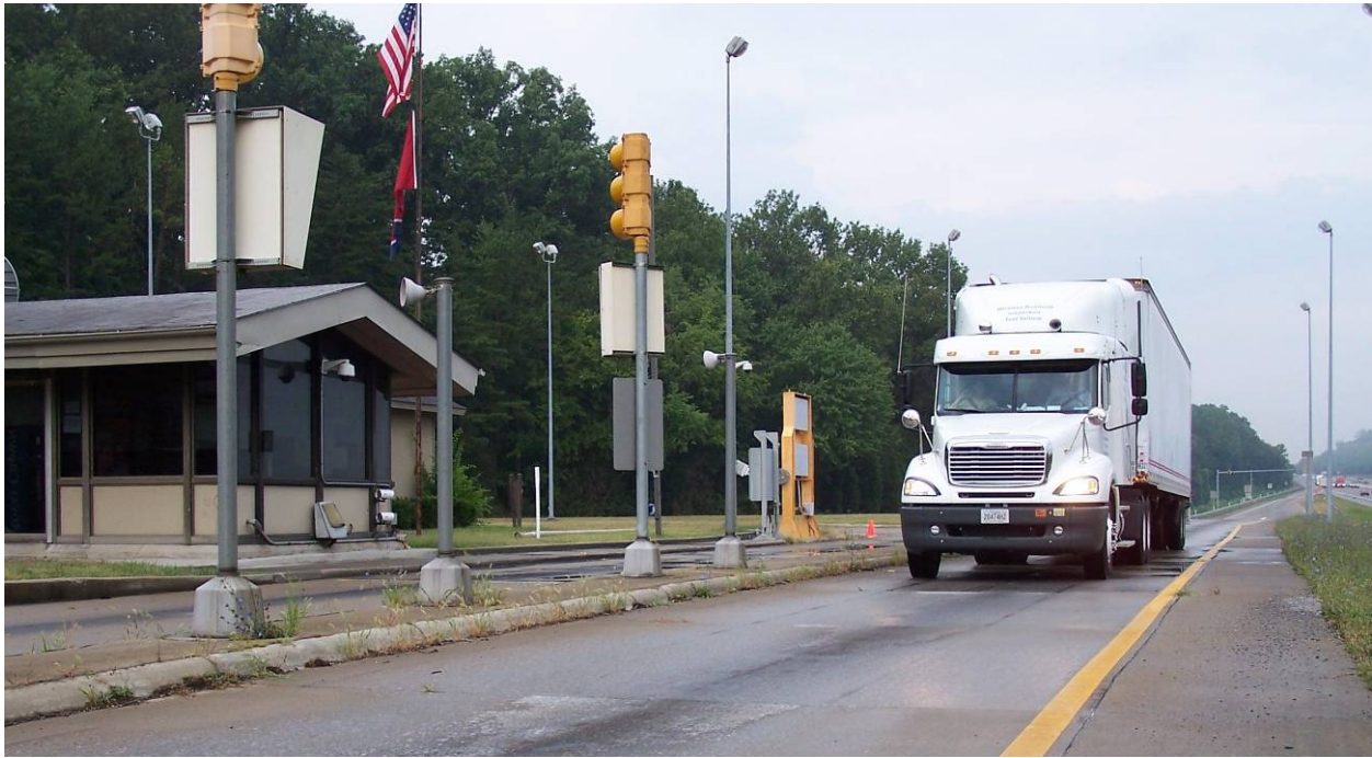
Figure 25. Location of Signs at Knox County Inspection Station
