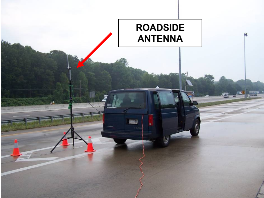
Figure 14. Roadside Unit at the Knox County Inspection Station
