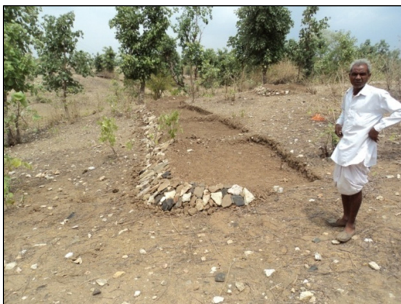
PHOTO 12: Soil and Water Conservation Work at Kamaliya
