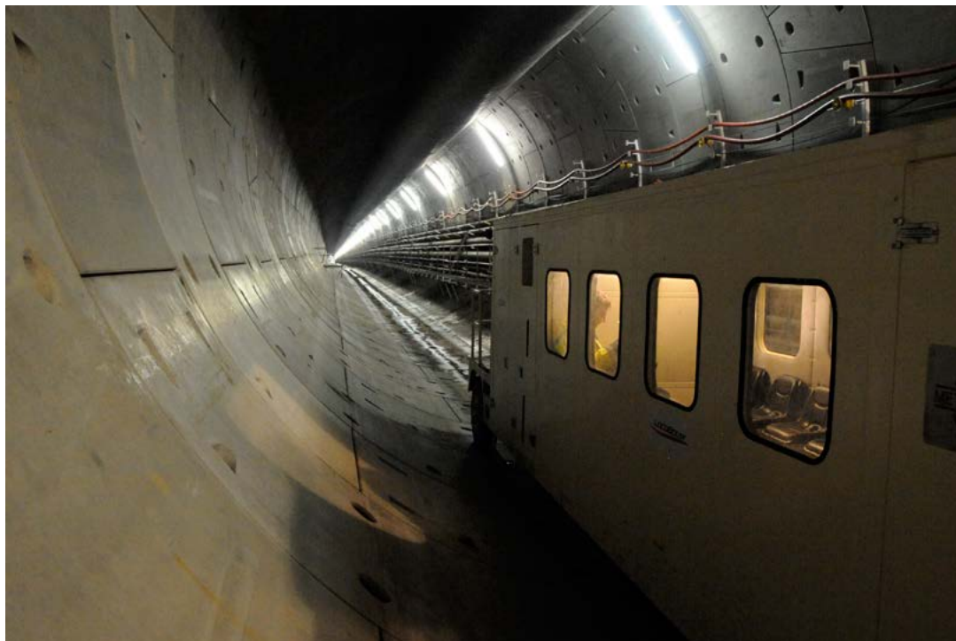
The Liefkenshoek rail tunnel connects the left and right banks of the Scheldt and offers more direct access to the hinterland.
