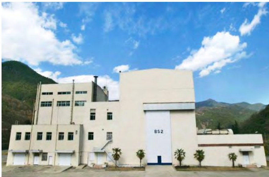
Figure 7-12 Non-Hazardous Operation Building (BS2)
