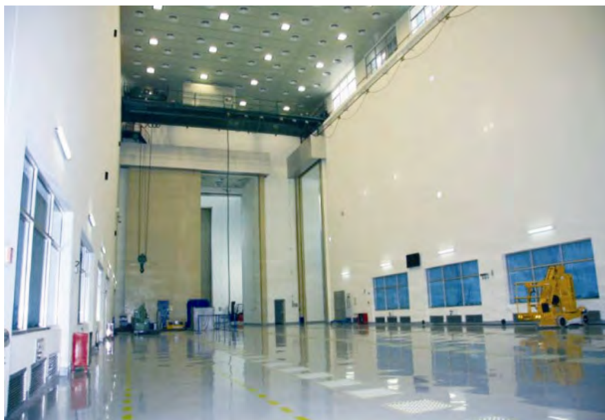
Figure 7-13 Non-Hazardous Operation Building (BS2)
