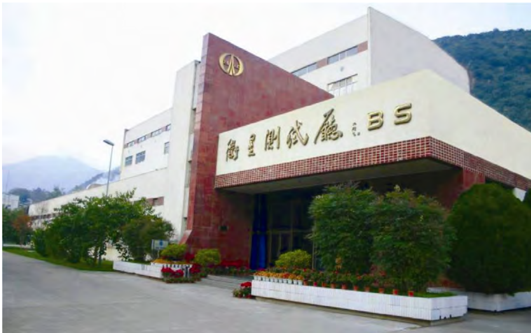
Figure 7-9 SC Processing Building (BS)
