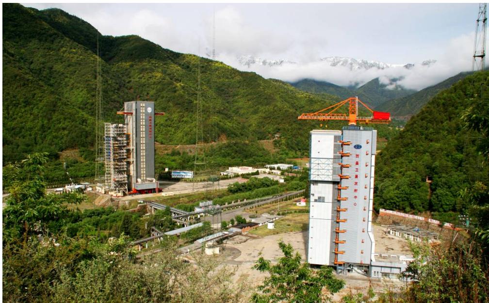
Figure 7-18 Two Launch Pads in XSLC (Left: LC-2; Right: LC-3)
