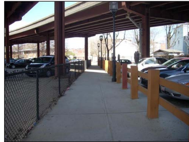
Photo 4: Walnut Street Walkway
