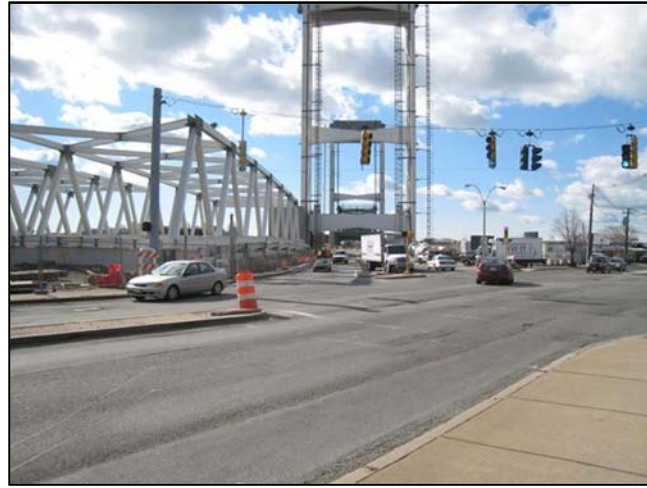
Photo 1: Eastern Avenue Intersection
