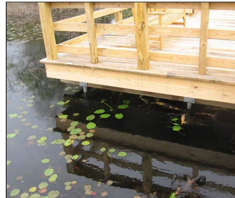
Design Precedent – Helical Screw Anchor Foundations
