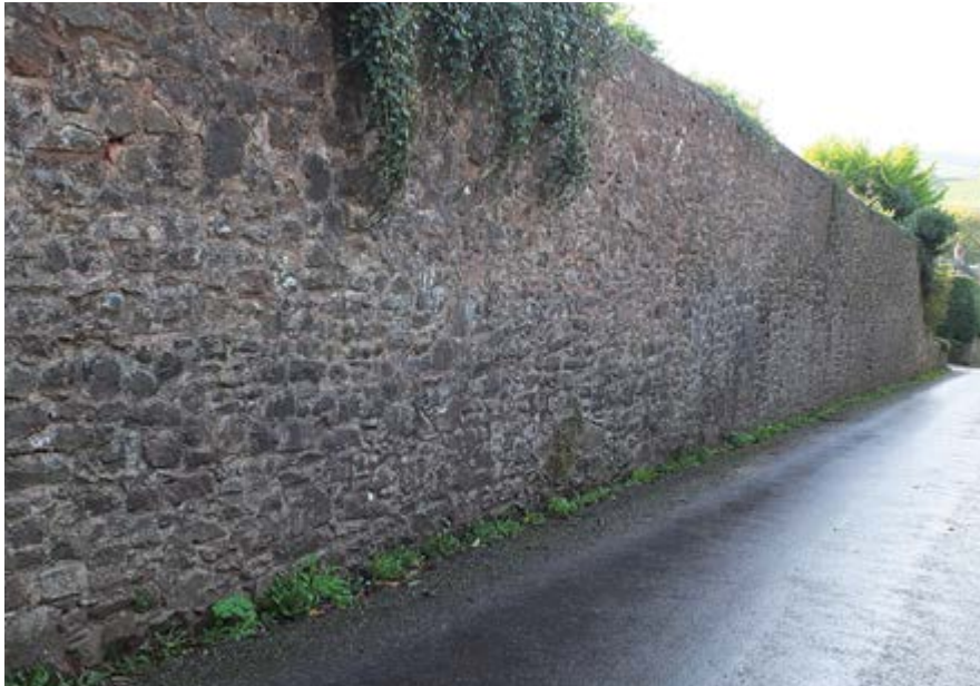
Fig 35 Boundary wall to Old Rectory
