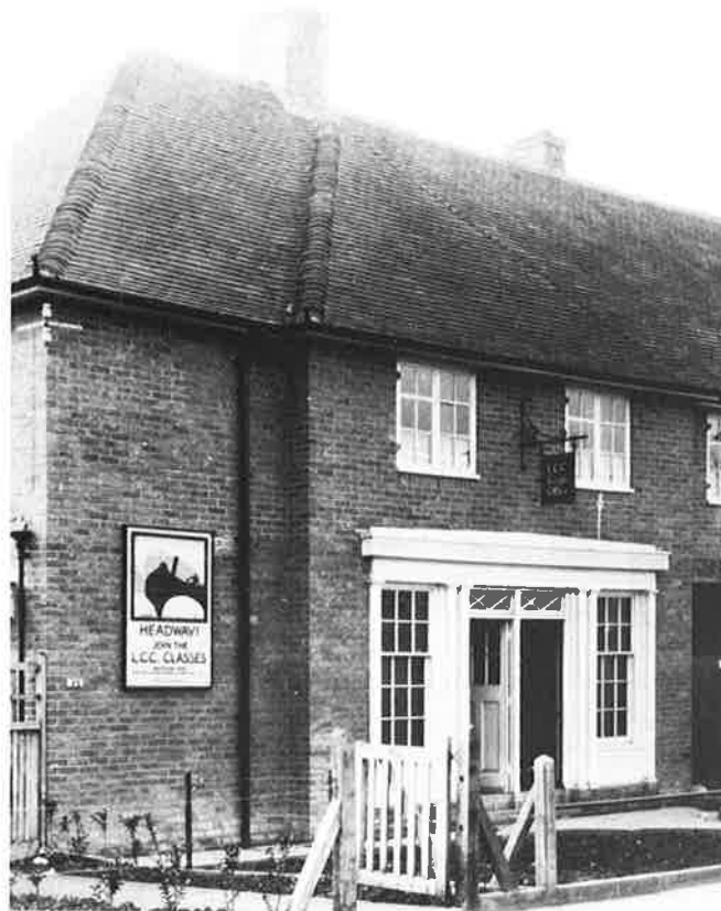
Downham Estate Office, Headcorn Road, 1927. Note LCC classes sign
