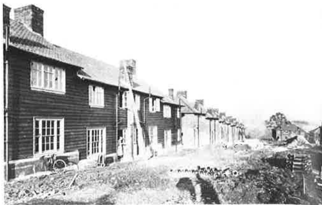
Watling Estate. Road 3, blocks 22/25. Building in progress, Nov. 1926
