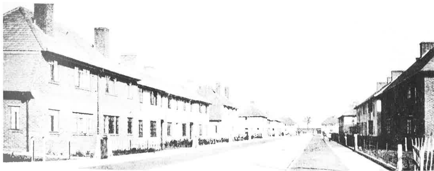
Alternate use of brick and white and coloured concrete, Becontree
