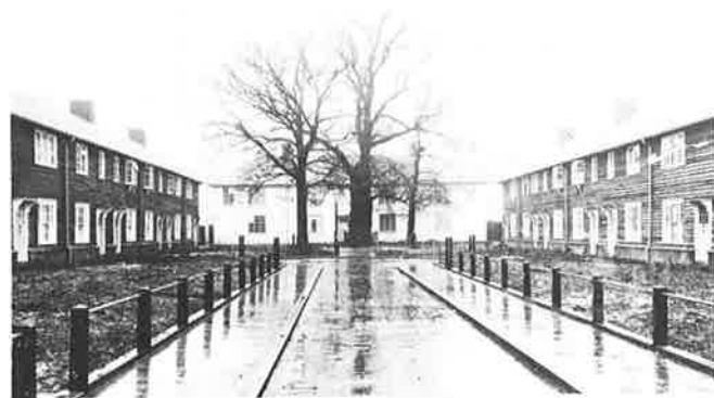
A typical cul de sac (banjo type) on the Watling Estate. Timber framed non-parlour and Atholl steel four roomed parlour houses, 1928
