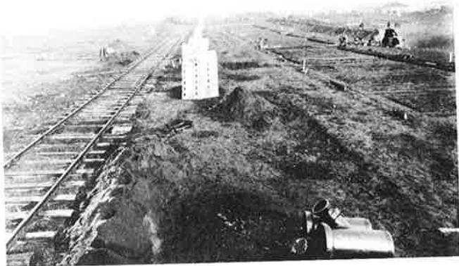
Becontree. Railway track to distribute materials to building plots.
