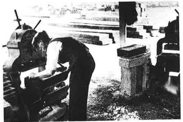
Pressing concrete blocks by hand, Becontree. Notice blocks curing in the background
