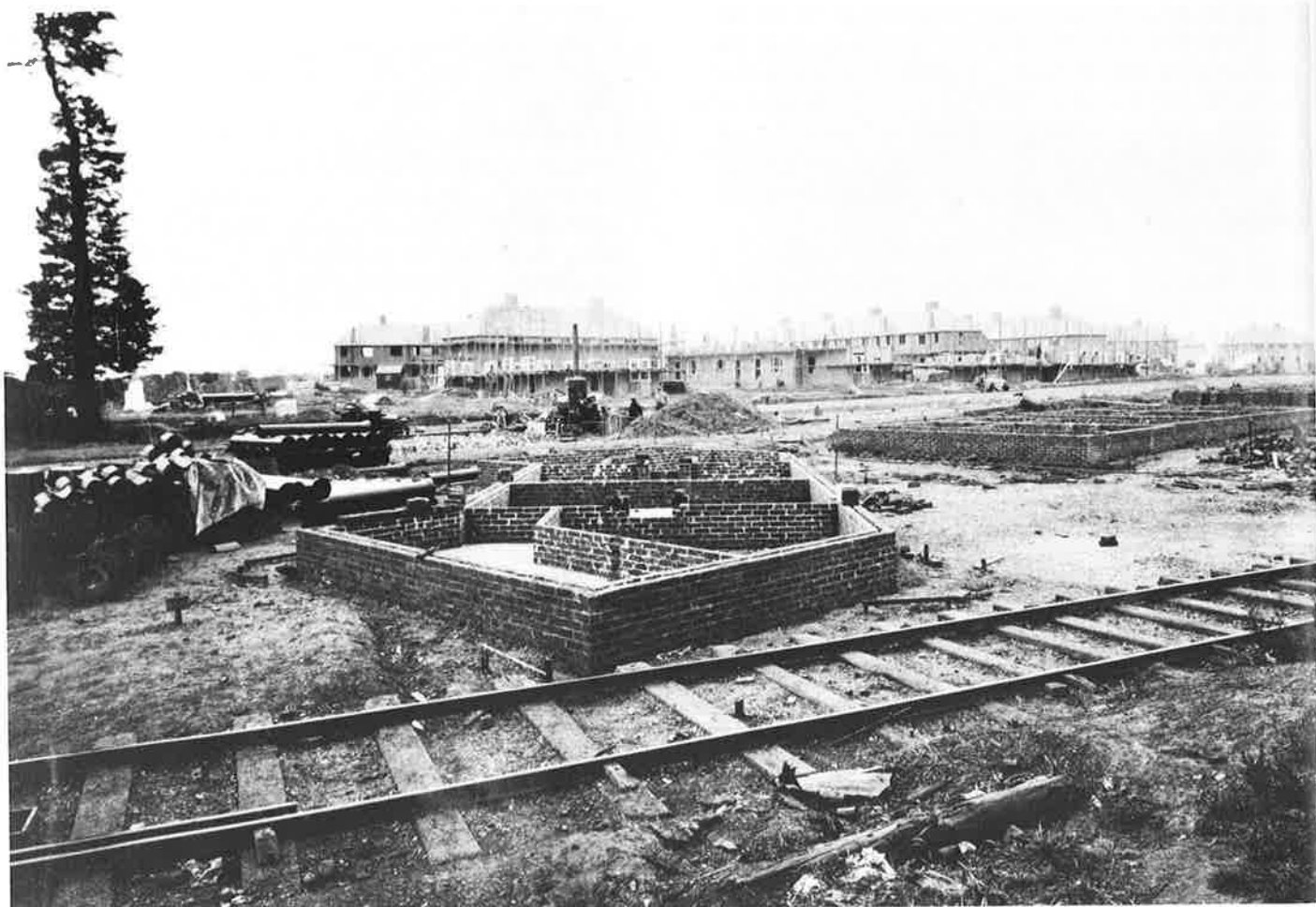
Becontree 1925. General view from 148 Langhorne Road showing foundation walls set out
