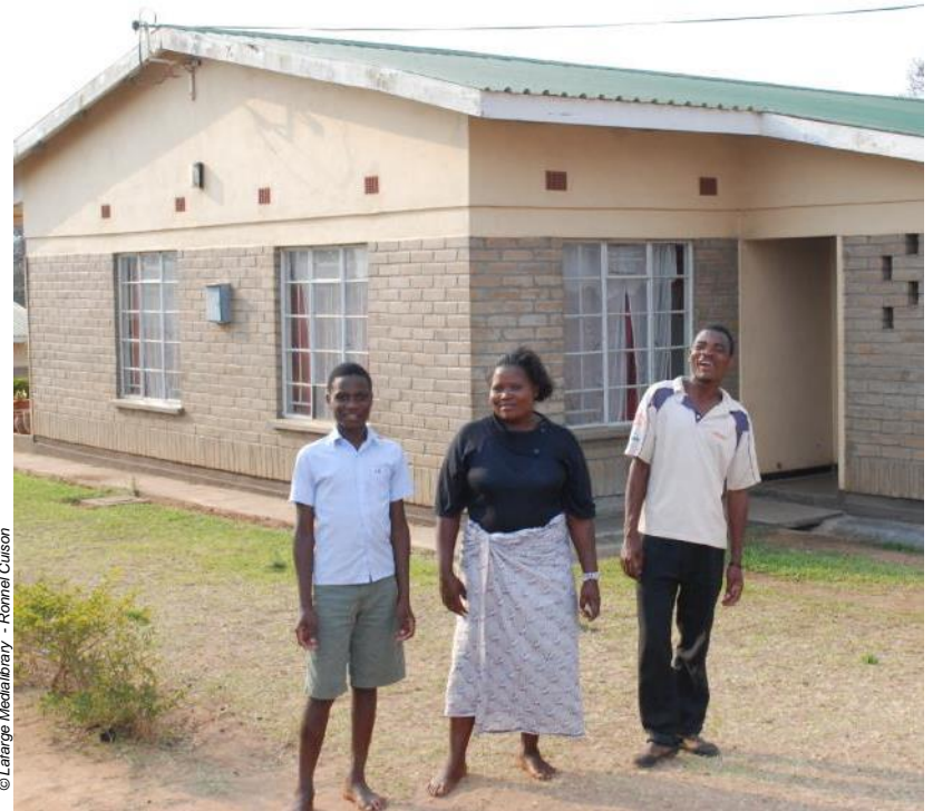
Malawi: A new « Earth and Cement » solution has been specifically formulated to manufacture soil-stabilized blocks, for affordable and green-friendly housing.
