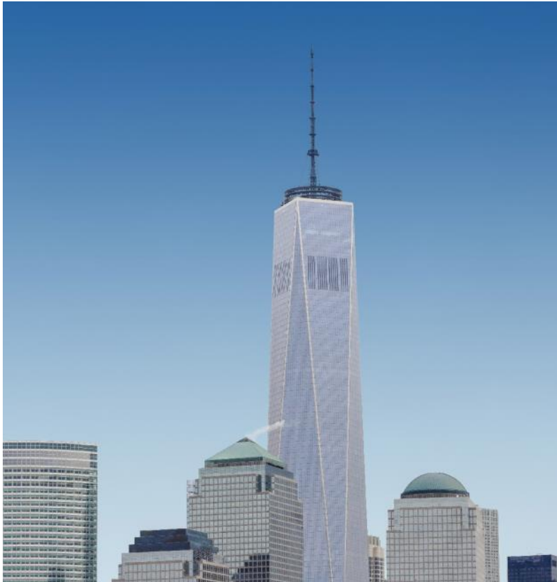
New York, USA: Lafarge has provided 150 000 m 3 of concrete used in the superstructure of the One World Trade Center in New York. This tower was designed to be the safest and most respectful commercial building in the world.
