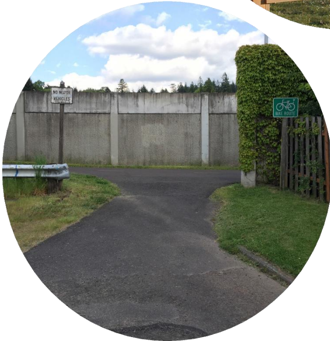
I-205 Multiuse Path access from Spencer Drive as it appears today
