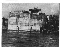
PHOENIX, a concrete blockhouse mounting AA guns, is pushed into place before being sunk as part of breakwater.
