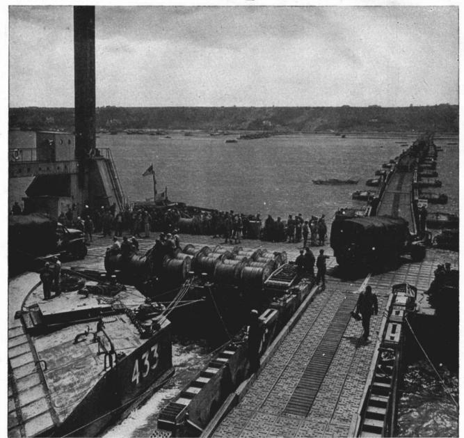
Supplies are unloaded at Loebnitz pier and roll ashore over pontoon bridgeway that falls and rises with tide.
