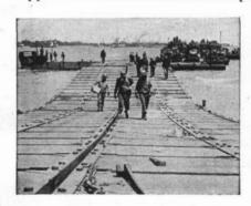
CAUSEWAY, one of several, slopes down from beach to floating pierbead for unloading landing craft.
