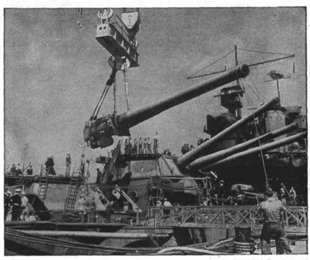
CHANGING WEAPONS: Giant crane moves worn 14-inch gun of veteran U. S. battleship to flat car during refitting operations at Bremerton Navy Yard where the BB was given armament with new linings.
