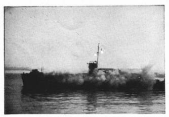
ROCKET-FIRING LCIs made their debut in 1944. Here one of them blasts enemy position on Leyte. Rockets were also used on other landing craft and on Navy aircraft during the past year.
