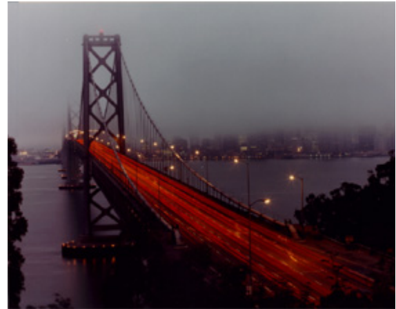
Personal income in the Bay Area is characterized by the largest discrepancy between high net earnings and low transfer payments. San Francisco Oakland Bay Bridge. Photo courtesy of CalTrans.
