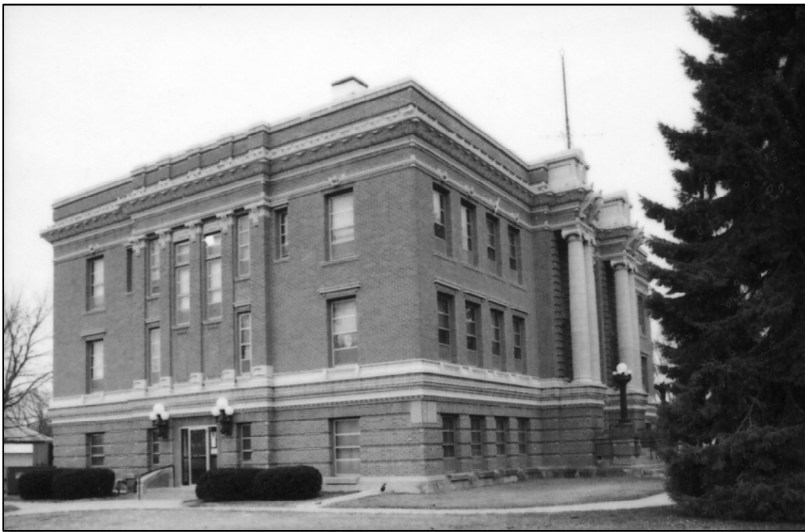
Looking southwest showing north and east facades Photo by BJB Long, Four Mile Research, 1989 (NSHS 8904/4:36)
