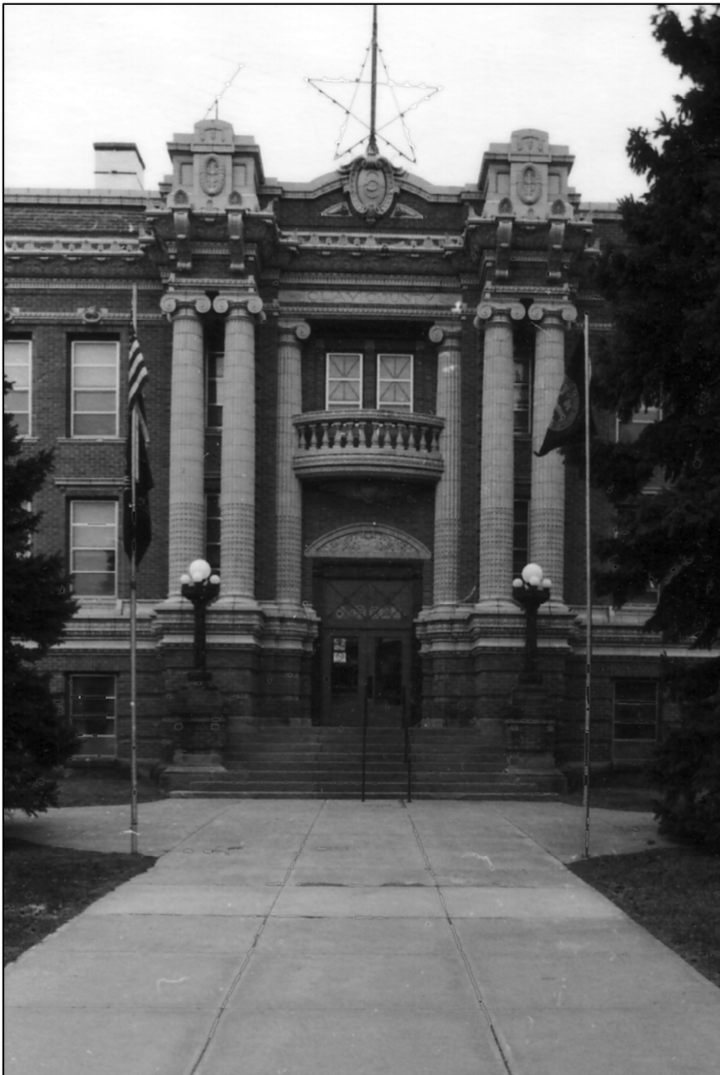
Looking south showing north entry pavilion & rich terra cotta detail Photo by BJB Long, Four Mile Research, 1989 (NSHS 8904/4:14)
