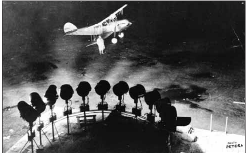
Flood light system used in the 1930s at Newark Airport.
