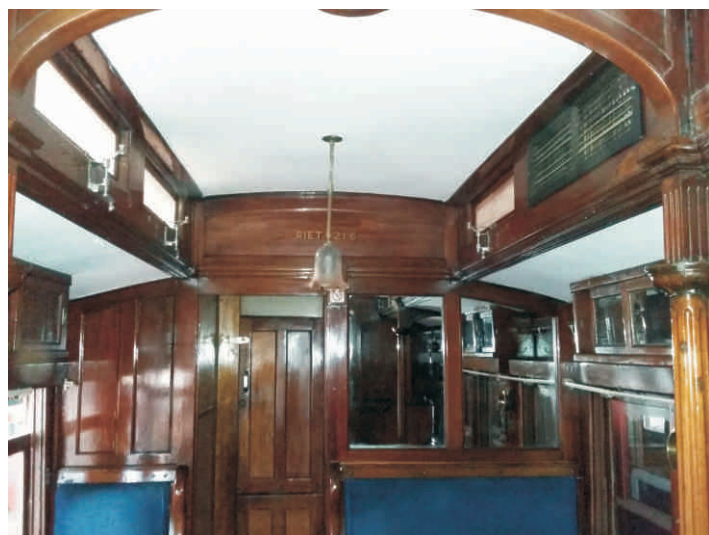
The interior of 218 during restoration.
