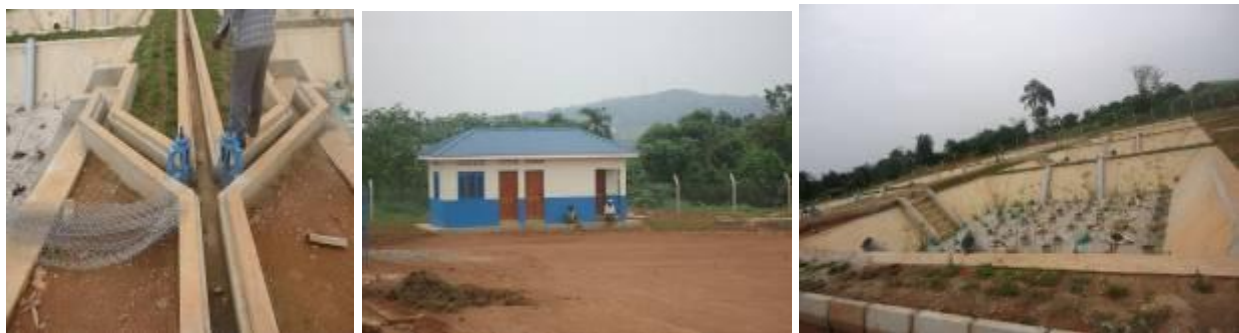
L-R: Sludge drainage channels with control valves installed; Guard house, store, toilet and a section of the compacted solid waste disposal site; Papyrus planted in one of the stabilization ponds, Mpigi district
