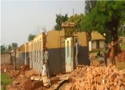
Ongoing renovation of the Male Ward at Masindi Hospital
