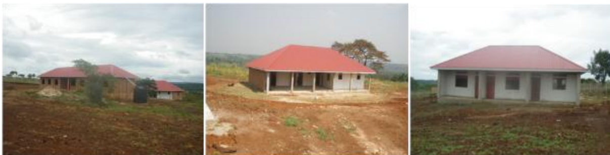
Left: The Maternity Ward, Middle: Outpatients Department, Left: Staff Quarter blocks at Nalutuntu Health Centre III in Mubende district
