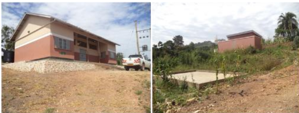
Left: Completed maize facility; Right: Drying slab and a bathroom facility in background in Mende sub-county, Wakiso district
