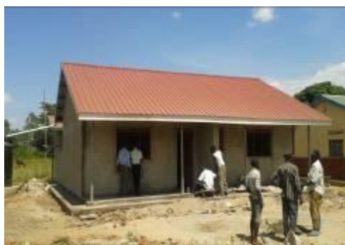
Construction of two-in-one staff house at Katira HC III, Budaka DLG
