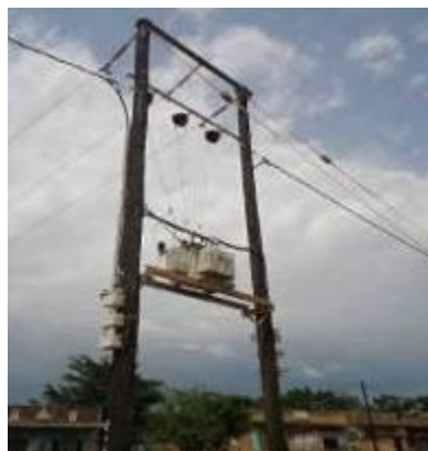
L-R: Completed stringing of Medium voltage line and transformer installation in Wabusana, Luwero district for Lot. 3
