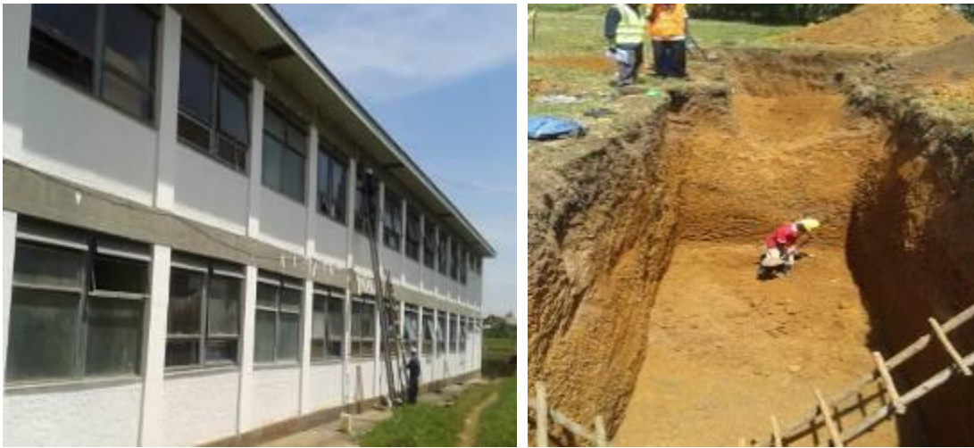
L-R: Ongoing painting at the maternity and children's ward and exaction of the septic tank at Bugiri hospital
