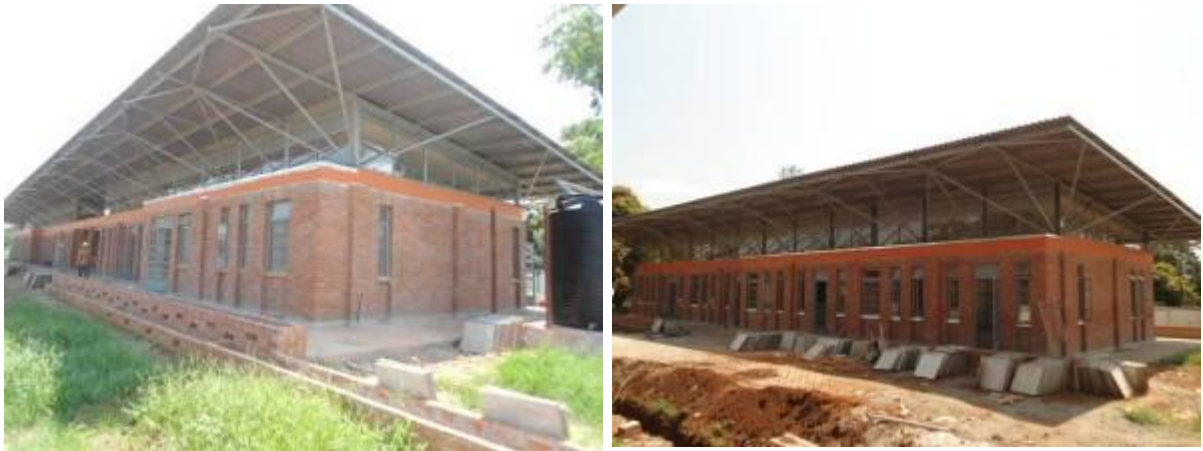
Left: The Resource centre, Right: One of the three lecture blocks constructed at Kaliro NTC
