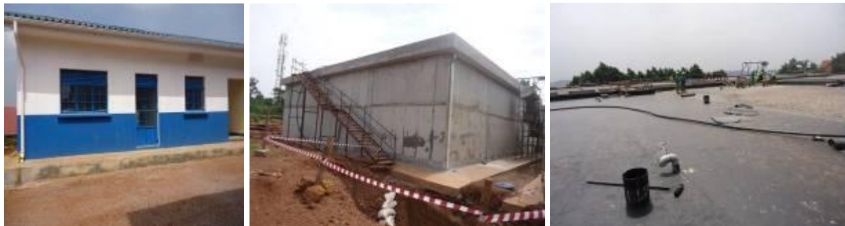
L-R: A section of the office building; One of the reservoir tanks; Placing bitumen on top of one of the tanks at Namasuba Hill
