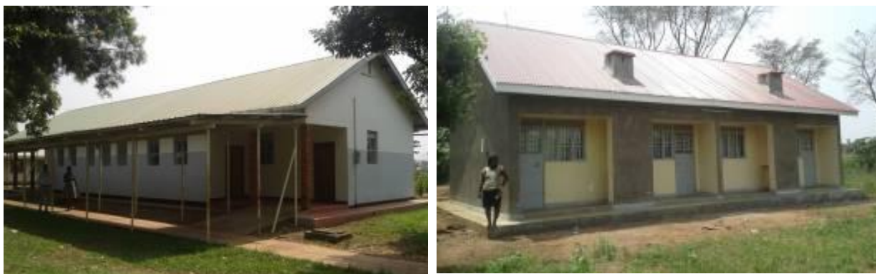
L-R: Renovated theatre at Kangulumira HCIV; Completed staff quarters at Buyobe HCII, Kayunga district
