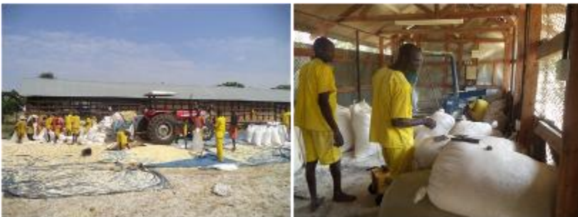
Left: One of the three repaired maize cribs; Left: Functional powered maize mill at Namalu Prison, Nakapiripit district
