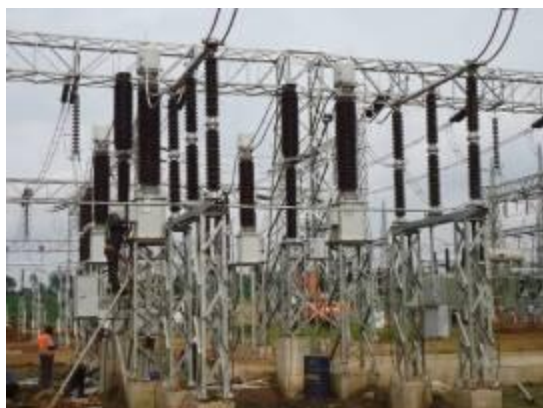
L-R: Finishes works on the electro-mechanical installations; completed line bays at Bujagali switchyard in Jinja district
