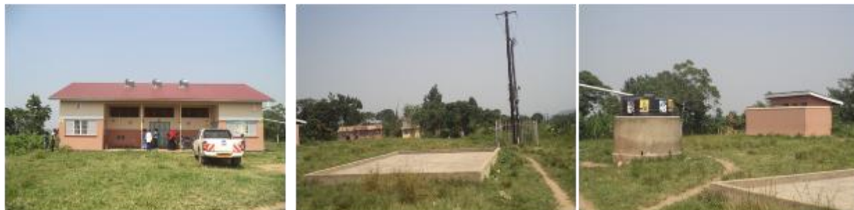
Left: Non-functional maize facility; Middle: Drying slab and grid connection in background: Right: 1,000 litre capacity water tank connected to bathroom facilities in Kibibi sub-county, Mpigi district
