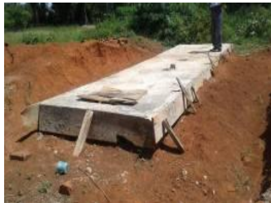
L-R: General ward under renovation and a four stance Pit latrine under construction at Iki-Iki HCIII, Budaka district
