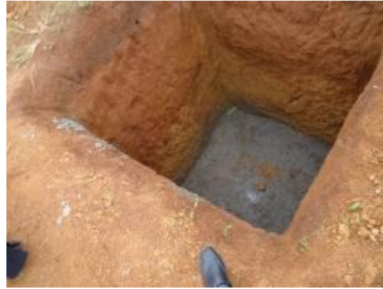
L-R: Poor quality aggregates dominated by dust that was used for Plain Concrete Cement (PCC); Completed PCC works in Lwela-Masaka
