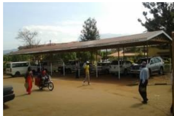
Nearly complete car shed at Mbale RRH
