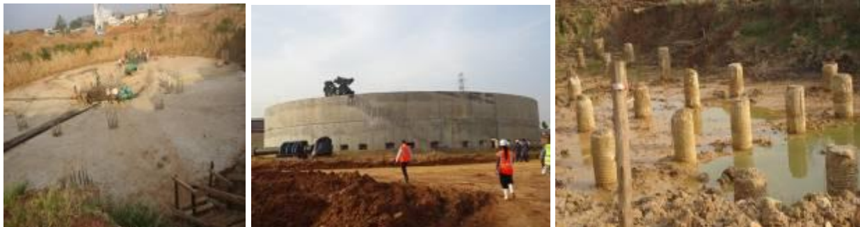
L-R: Sedimentation tank base; Trickling filter; Sedimentation tank pile foundations at Bugolobi, Kampala district
