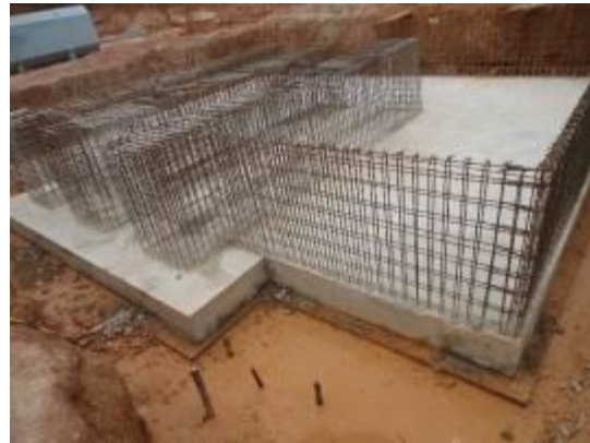
L-R: Poor quality aggregates dominated by dust that was used for Plain Concrete Cement (PCC); Completed PCC works in Lwela-Masaka
