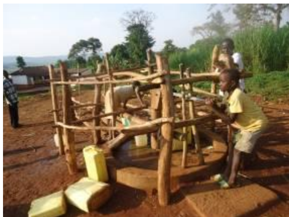
Jinja district: Nabilama rehabilitated borehole in Basude sub-county
