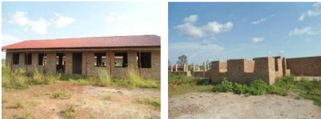
Left: A two classroom block, Right: An administration block left incomplete at Engineer Kauliza Kasadha Technical Institute – Bugiri District
