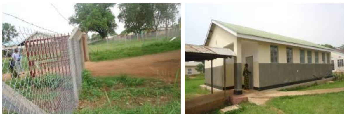
L-R: Fencing works and rehabilitated theatre at Amach HCIV, Lira district
