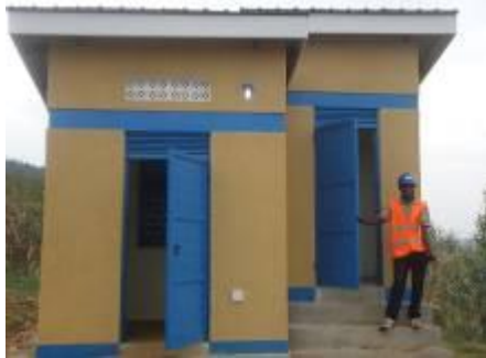
L-R: Grid power and pump house for pump station 2; Chlorine house; Ecosan toilet and guard house at pump station 1 in Jinja district
