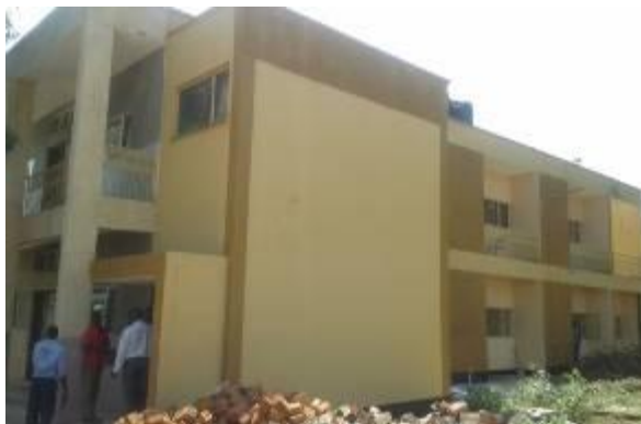
Renovation works at the Interns Mess at Mbale RRH
