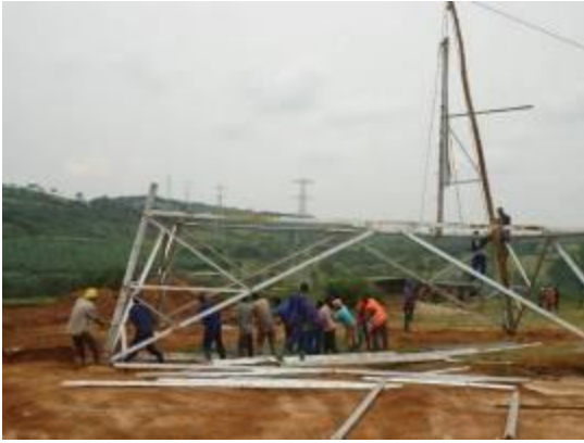
L- R: Tower erection ongoing; Completed tower erection in Mirama for the NELSAP project
