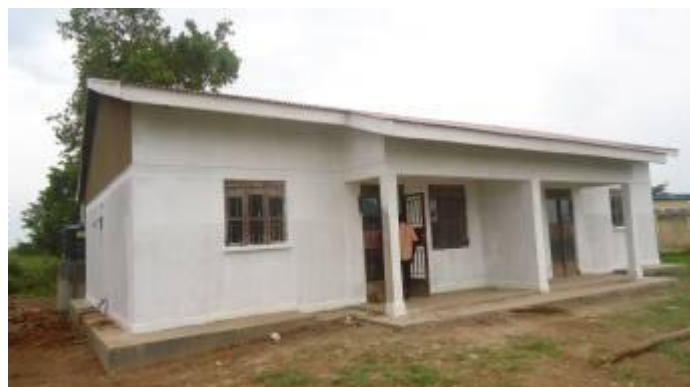
Semi-detached staff house under construction at Acao HCII, Apc district
