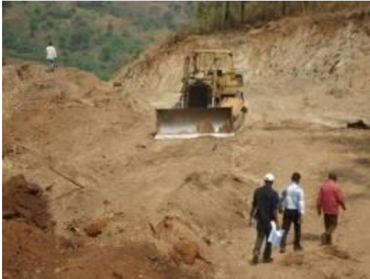
L-R: Ongoing excavation works; Cut for filling in some sections on the road under construction at Nyagak III, HPP in Paidha Town Council
