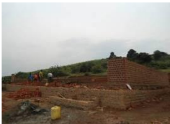
Construction of the multipurpose hall ongoing at Kifamba Comprehensive S.S. in Rakai district
