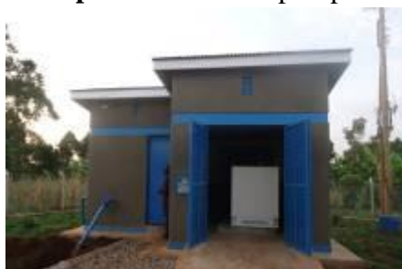
Pump house at pump station 1 in Lwanda village, Luuka district
