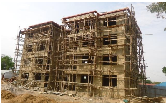
Construction of two bedroomed staff quarters at Lira RRH
