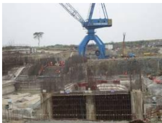
L-R: Form, steel and other civil works ongoing at the powerhouse site at Isimba Hydro power plant in Kayunga district
