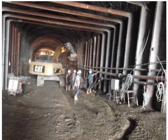
Left: Ongoing excavations Right: Construction works on the Escape/ Ventilation Tunnel on Karuma HPP
