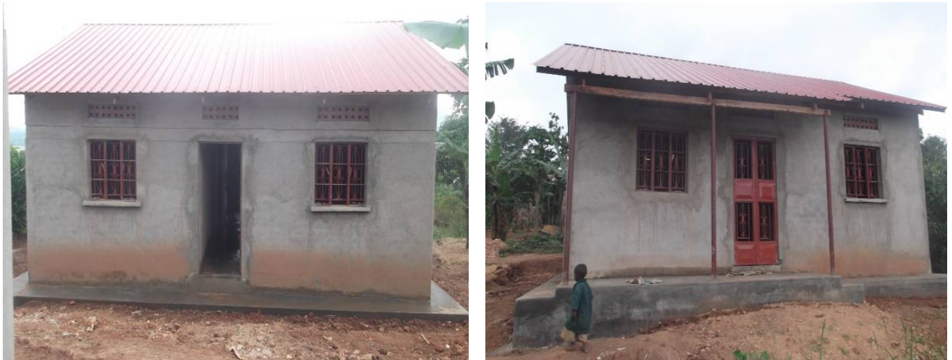
Resettlement houses for PDPs on the Kawanda- Masaka transmission line.
