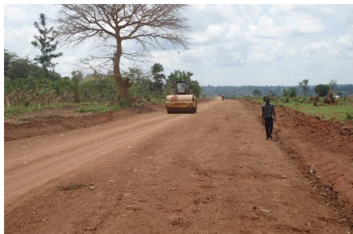
Right: Levelling of access road
