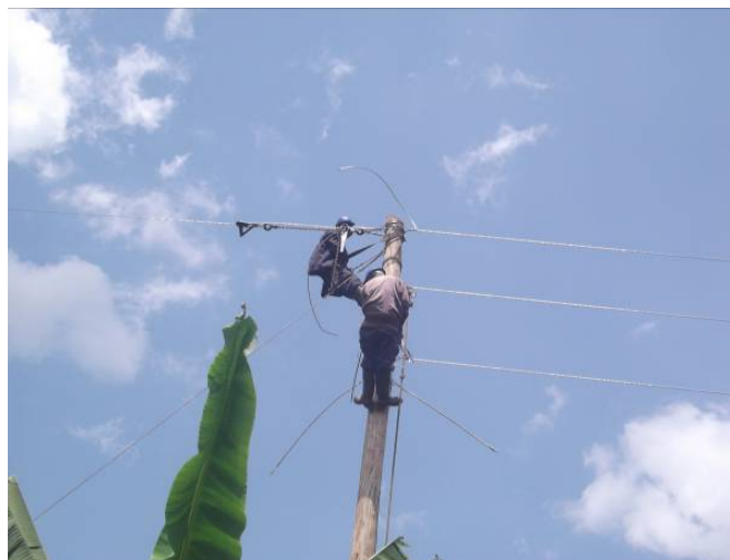
L-R: Completed Pole erection in Kasambya Subcounty; Ongoing stringing works in Kayunga District
