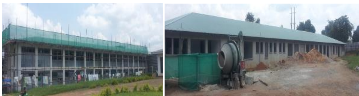
Ongoing renovation works on the existing T-block at Kiryandongo Hospital
