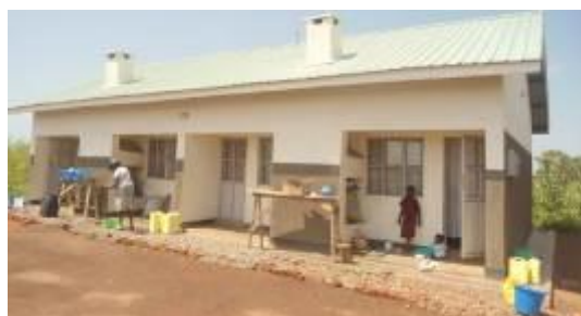
Four-in-one staff house at Lalogi HC IV, Gem Parish, Lalogi Sub County in Gulu District
