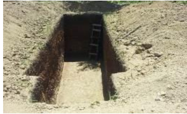
Left - OPD at Tumangu HCII, right is the excavated drainable pit latrine
