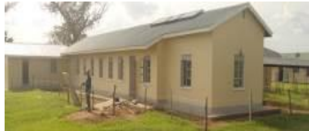
General ward at Awach HC IV in Gulu District under renovation
