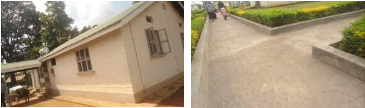
Renovated Interns mess (left) and newly constructed walk ways on the (right)
