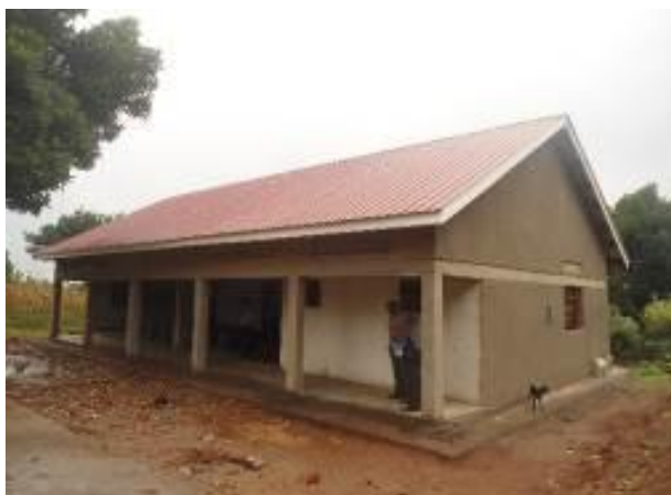
OPD under construction at Mpugwe HCIII
