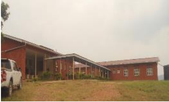
Newly constructed Kisozi HC III
