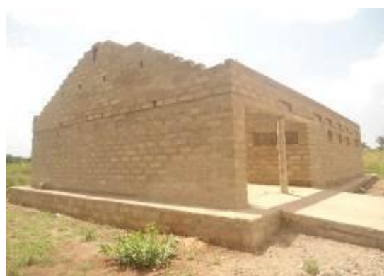
Construction of OPD at OMolodyang HCII
