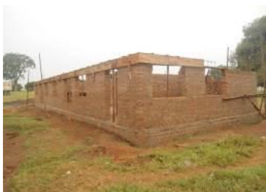
Theatre at Kumi HCIV under construction
