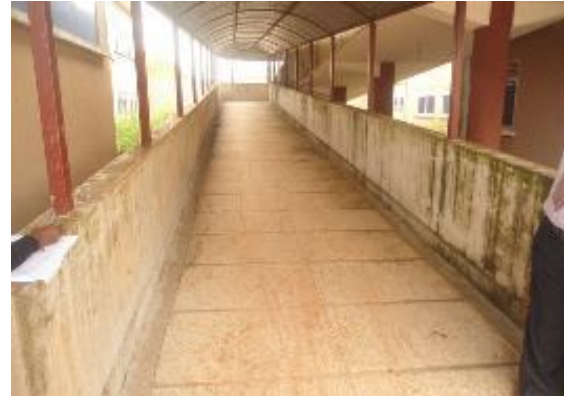
Newly constructed Private wing at Jinja RRH (Left) Walk way of the private wing with green algae growing on the walls
