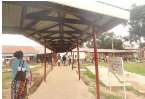
Newly constructed sheltered walkway at Soroti RRR
