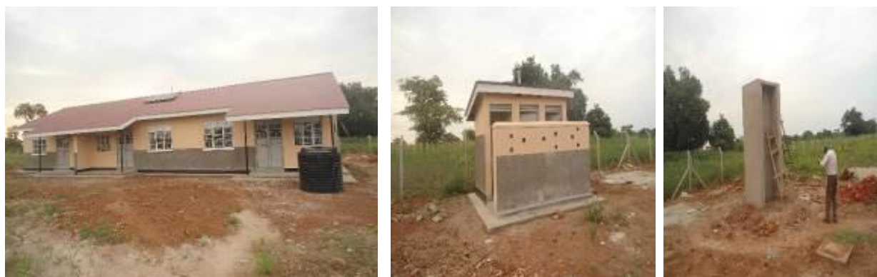
Completed staff house, Pit latrine and tank stand Tiriri HCIV
