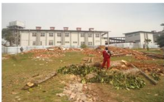
Site clearance for the maternity ward complex
