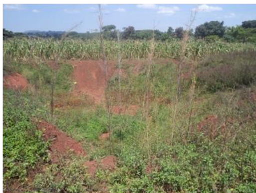
Unattended burrow pit that was not filled and leveled by the road side in Bugiri district
