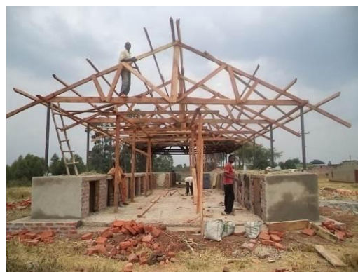
Ongoing construction works of Kyarushozi market in Kyenjojo district
