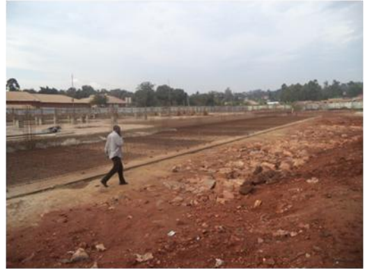
Foundation level of the construction works at Busega market
