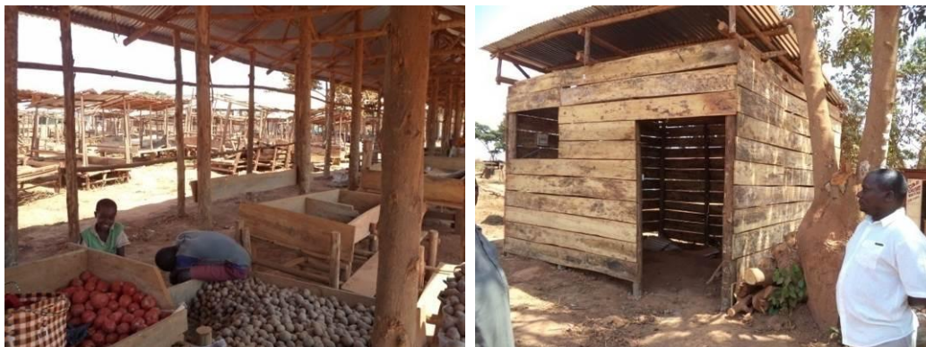
Left: Completed market structures; Right: Market Coordination Offices
