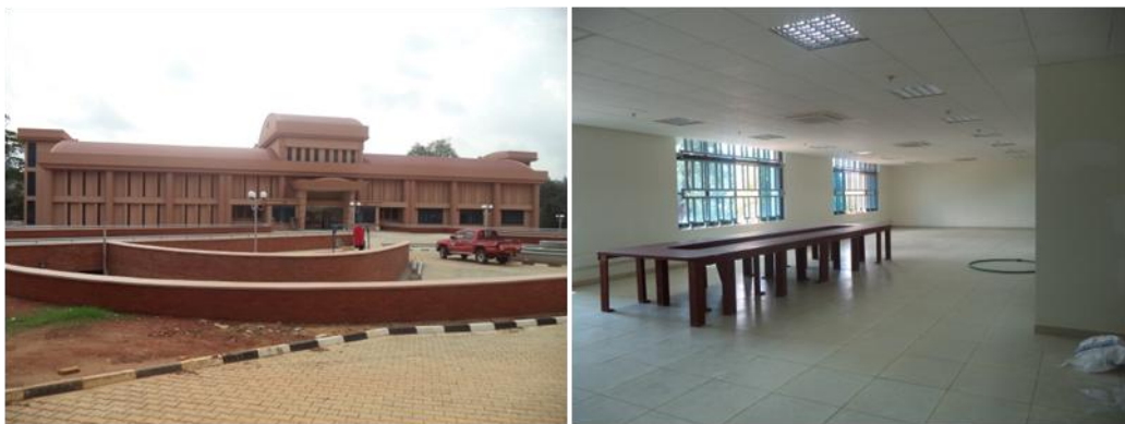
Left: front view of NARC building; right: archives room for storage of records from local governments in premises at Nakasero, Kampala
