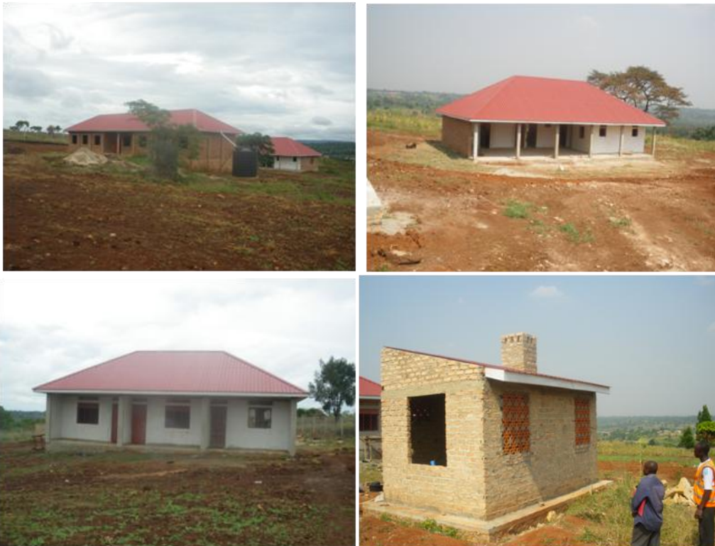
Top left: Front view of the Maternity Ward; top right: Front view of Outpatients Department; bottom left: Staff Quarter block; bottom right: unfinished kitchen for staff quarters in Mubende district
