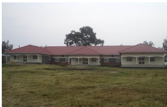
Completed Youth Centre in Kabarole district
