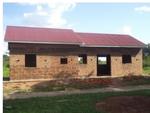
Roofed health centre in Kumi Sub-County
