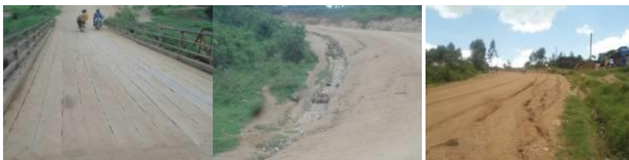
Timber decking on Katete bridge (left); open drainage channel with rubbish (centre); and gulleys forming on the road surface alongside the drainage. (right) on Rwizi Lane.
