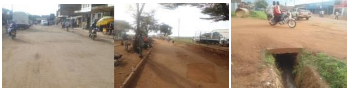
Stripping of surface on Togore Road West (left); Pot holes appearing on Obuya Lane (centre); and the newly installed box culvert on Park Lane. (right)
