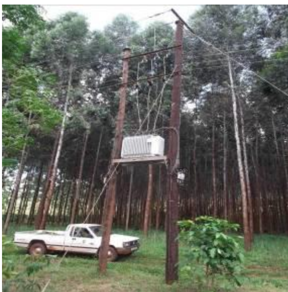
315KVATransformer on the Bujwaha-Bulyango line and Bukwiri-Kyankwanzi line
