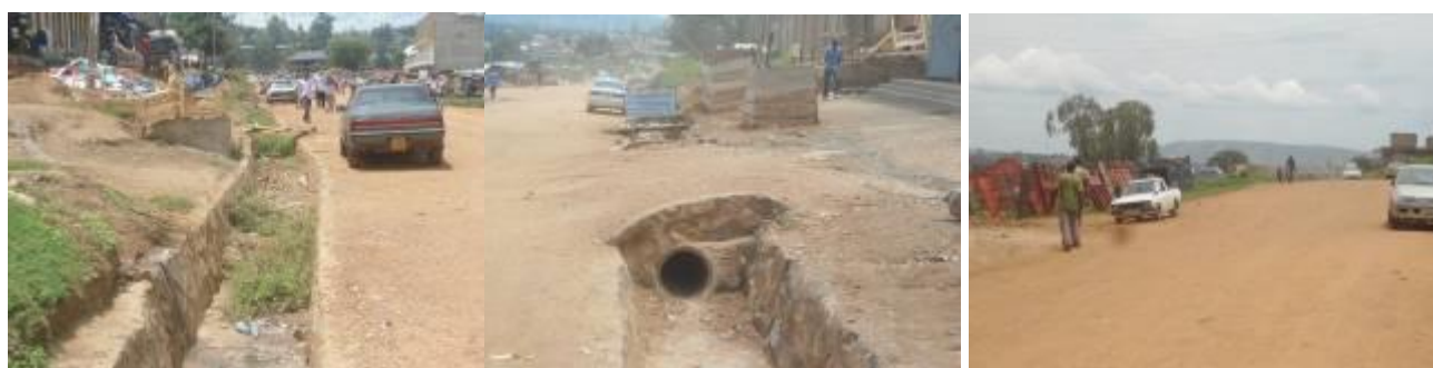
An open channel that is silting due to rubbish dumped in it. (left); A 600mm culvert line installed. (centre); The well graded, gravelled and shaped road surface. (right) on Major Victor Bwana road
