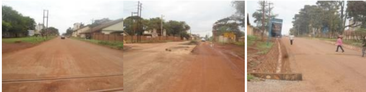
Completed section of the road at Railway crossing (left); Junction with Factory road with unfinished reinforced concrete works (centre); and stone pitched side drain works (right)
