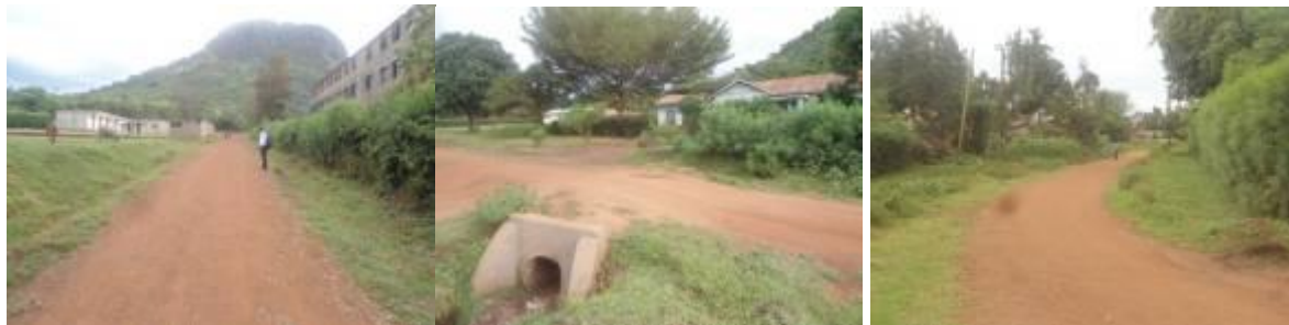
Well graded and gravelled 100m Access road (left); A newly installed culvert on Bukedi road. Note the depression at the far end of the culvert line which indicates a broken culvert. (centre); Hyena drive (right)
