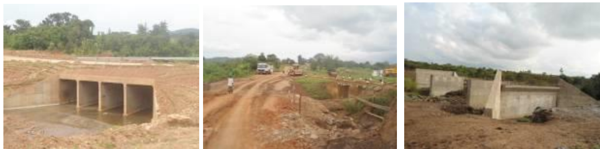
(Left): Completed Amua box culvert with guard rails installed; (centre); Completion of diversion works for Ebikwa box culvert works; (right) Incomplete Irei Bridge works with no deck.
