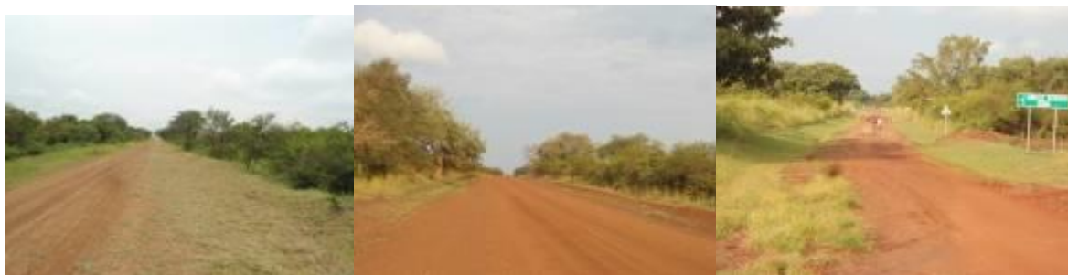
A graded section of MoyoObongi road where slashing of the road side was ongoing (left); A regavelled section of LaropiAyugi road. (centre); A graded section of DzaipiBibia road whose road surface was defecting due to poor compaction. (right)
