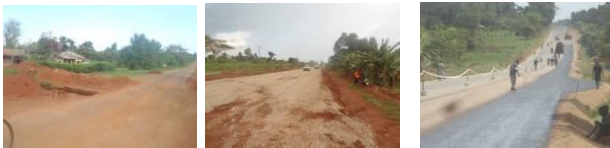
(Left); Section of the road where excavation for a culvert was ongoing with no safety precautions taken to warn the passing traffic and pedestrians. (Centre); A section of the road sub base that is undergoing mechanical stabilisation. (Right); A section near the junction to Namasagali undergoing base priming.
