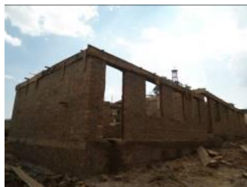
A three classroom block at whole plate level and a 2 classroom block at ring bim level at St.Thomas Bazadde P/S Bweyogerere
