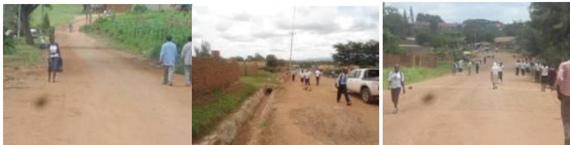
Graded section of Nkonkojeru Court road (left); Drainage works along Kakungulu drive (centre); and completed first seal of DBSD on Kakungulu drive (right)
