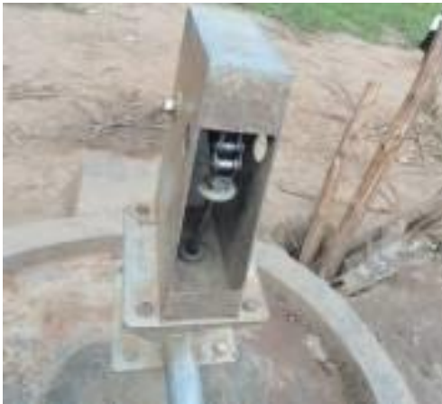
Vandalised BH pumphead at Kanani Buwama S/C.
