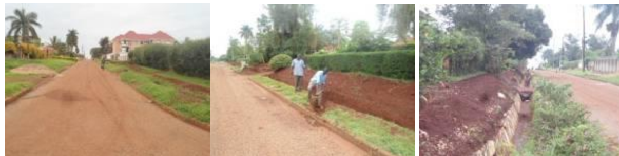
First bitumen seal (left); Excavation of side drain (centre); and stone pitching of side drain (right) along Madhvani road
