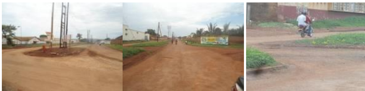
Concrete and second seal work at the Factory road junction (left); End of second seal works near Nile Ply (centre); and stripped surface in the island caused by heavy truck turning near Nile Ply (right)
