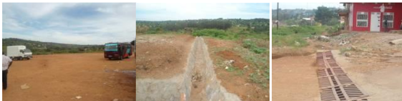
Stabilised murram that was provided for the lorry (left); Surface drainage works around the lorry park. (centre); Drainage channel along Ssesse street.
