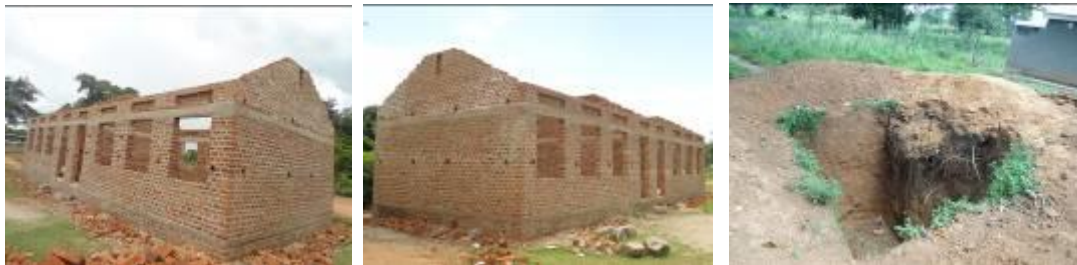
The 2 blocks each with 2 classrooms at whole plate level and the 2-stance VIP pit latrine at excavation level at Bugwe P/S
