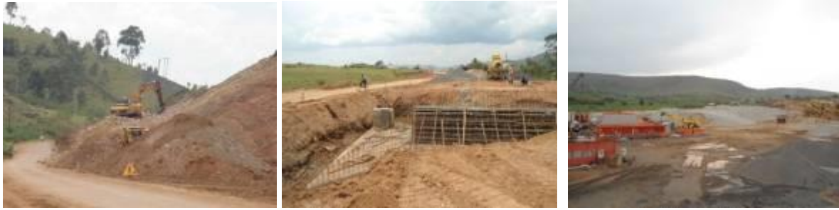
(Left): Rock excavation works along slopes; (centre); Construction of a concrete box culvert across the road at Km 67+800; (right) the stone quarry that is already in production of aggregates.
