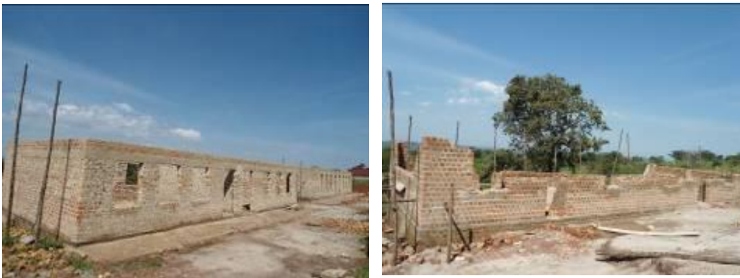
The 2 classroom blocks at ring bim level and the teachers' house at window level at Butoloogo Seed S.S
