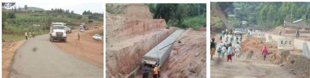
(Left): Base course works ongoing at Km 98+650; (centre); Installation of a 1.5m by 1m high culvert crossing at Km 100+488; (right) filling of embankment. Take note of the safety precaution taken by the contractor for the traffic using the project road.
