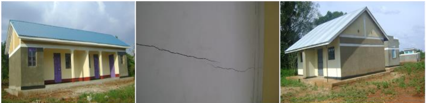
Kamuli district PHC development: staff house at Luzinga HCII (left); cracked ceiling in staff house at Luzinga HCII (centre); staff house at Namaira HCII (right)
