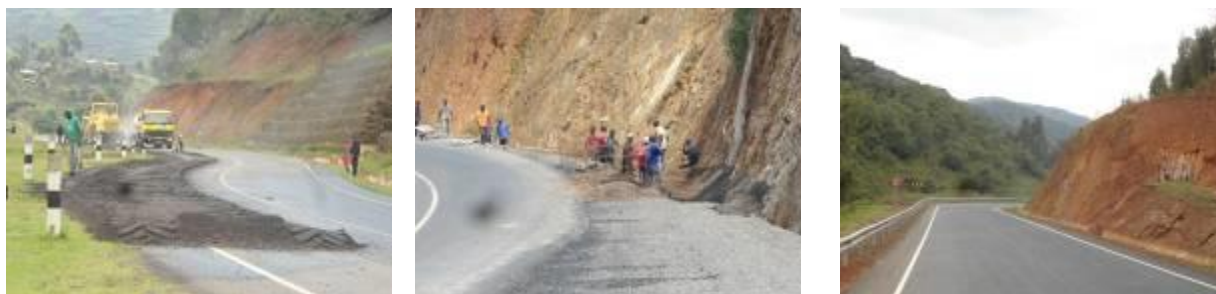
(Left); Completed section of the road where scarifying was ongoing. (Centre): Construction of a concrete line open drain. A section of the road at Km 8+300 yet to be surface dressed. (Right); Completed section of the road with the centre line not yet marked..
