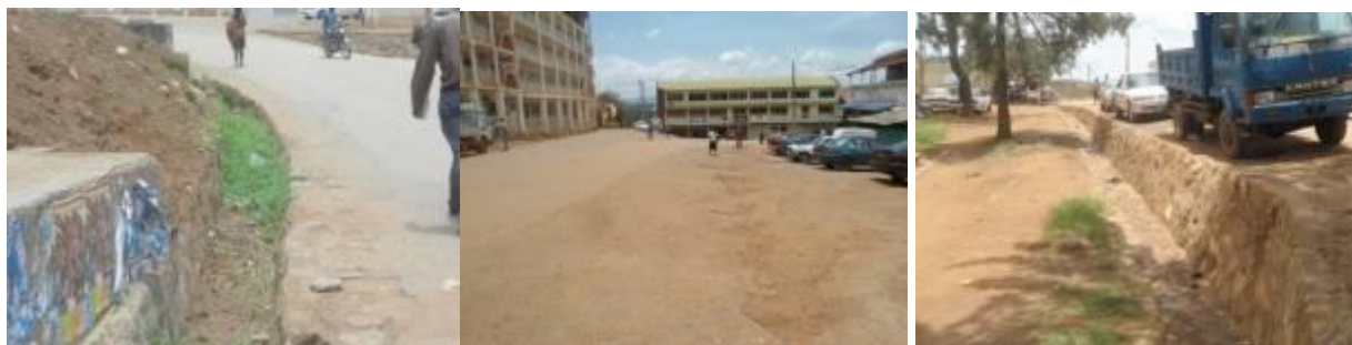
Silting in an open channel (left); sealed road shoulder (centre); and the 100m open drainage protected with stone pitching. (right) along Bananuka drive.
