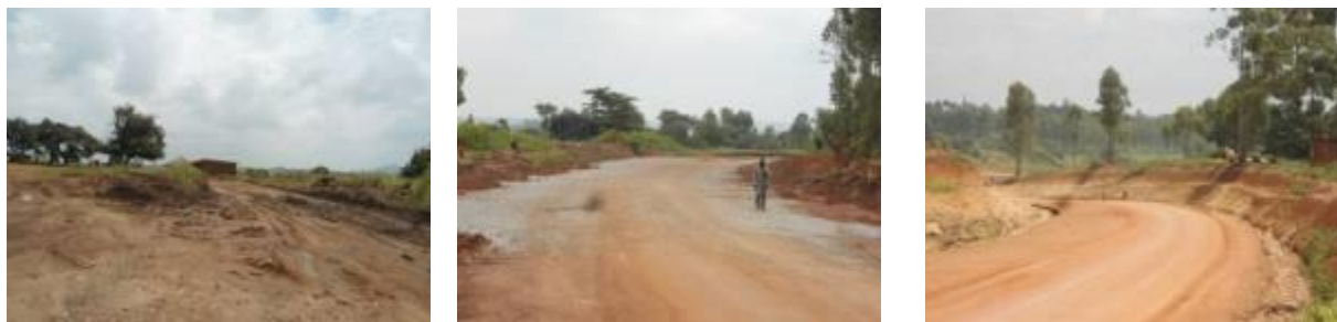
(Left); A section of the road at Km 61+930 where compensation issues have hindered clearing works. A grave and a house remain in the project area. (Centre): A section at Km 59 that is being maintained especially for heavy traffic that is using the road. (Right); Section of the road at Km 41 where the road has been cut to reduce on the gradient and subgrade works have been completed.
