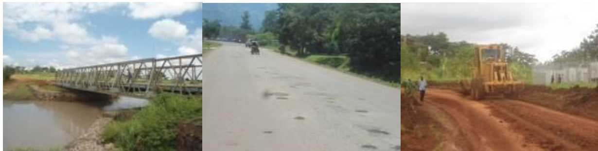
Kite –Kawanone bailey bridge (left); Section of SironkoMuyembeKapchorwa road where patching works were done but potholes are still coming up. (centre); Grading works ongoing on MbaleBufumbo road. (right)
