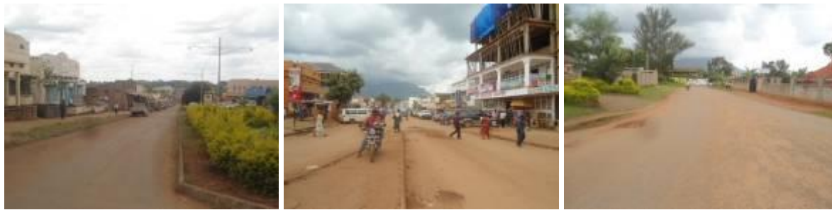
Parts of Naboa road and at the end that have the chippings stripped off (left and right) and potholes have developed before the hand over of the road at Km 0+000 (Centre)
