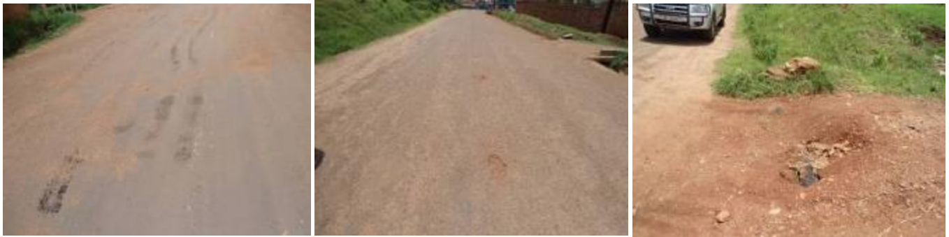
A section of Bweyogere park bleeding roads, potholes, failed culverts and incomplete drainage
