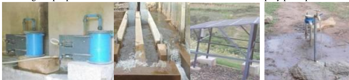
The Chemical doser Unit, the Gabion protection at intake, the solar panels and tap with water running (Tororo-Manafwa GFS)
