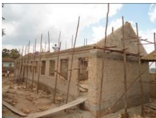
A three classroom block at whole plate level and a 2 classroom block at ring bim level at St.Thomas Bazadde P/S Bweyogerere
