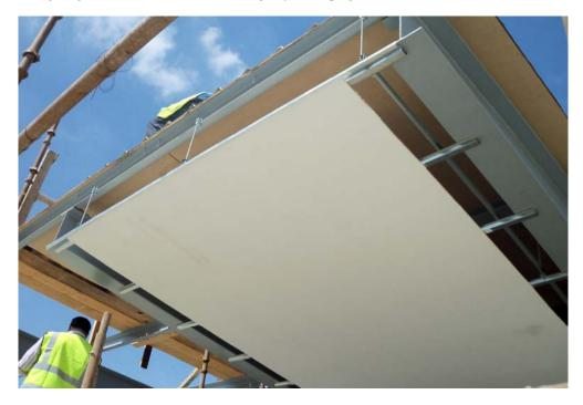
Fig. 4: Using Magnesium oxide boards supporting metal frame.
