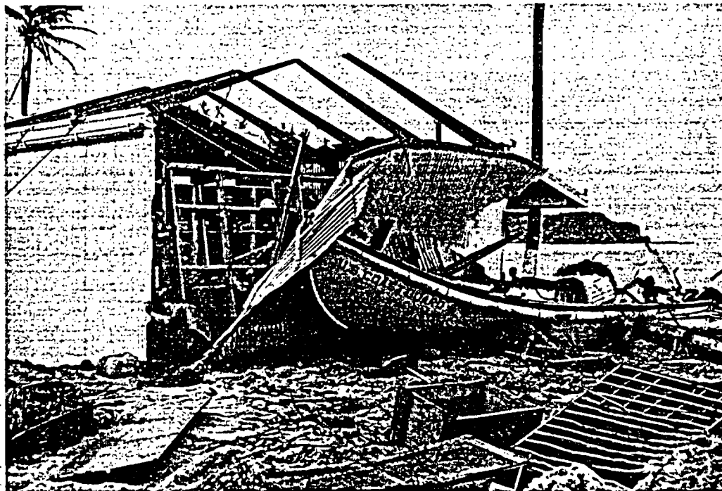
DAMAGE TO BUILDING AND BOAT CAUSED BY ELLEN, 9 DECEMBER 1961. (OFFICIAL NAVY PHOTO)
