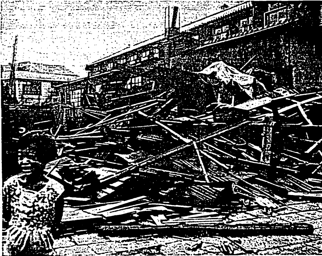
THIS RUBBLE WAS A BUILDING BEFORE PAMELA STRUCK TAIWAN. SEPTEMBER 1961. (PACIFIC STARS AND STRIPES)
