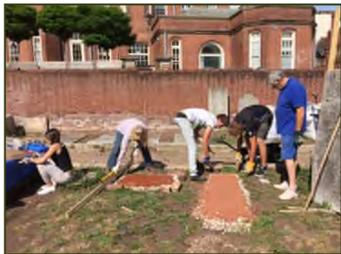
Volunteers creating drainage plinths to raise the memorial stones off the soil surface.
