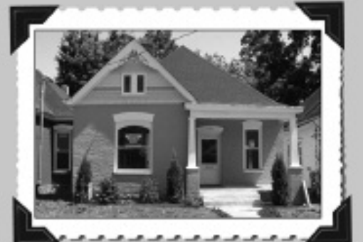
416 Johnson Avenue – After
