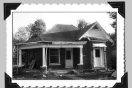
422 Johnson Avenue – Before
