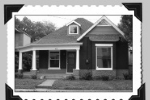
422 Johnson Avenue – After
