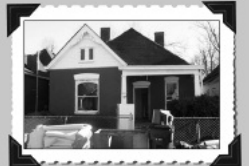
416 Johnson Avenue – Before
