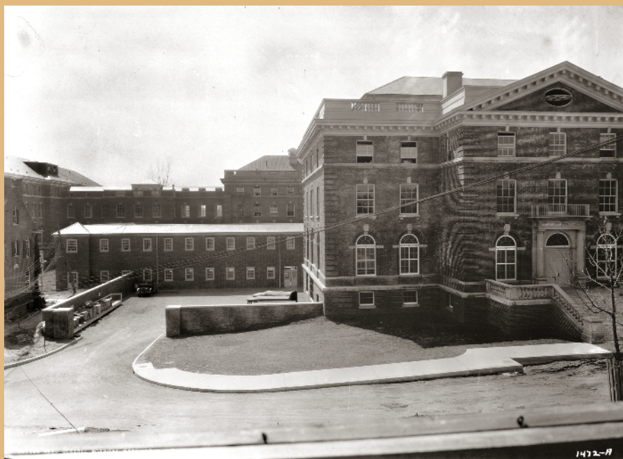
1927, Entrance to Kitchen Area; Right: first floor, Mess II; second floor, Library; third floor; EENT Wards.
