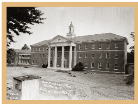
1931, First Construction at Delano Hall
