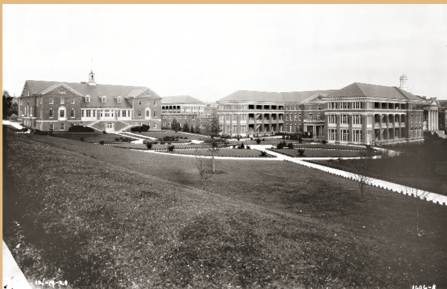
1929, New Red Cross Building and West Wing Main Building
