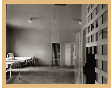
Guard House, Interior View
