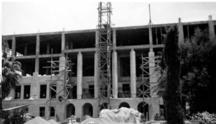
Building the 1938 Capitol Addition.
