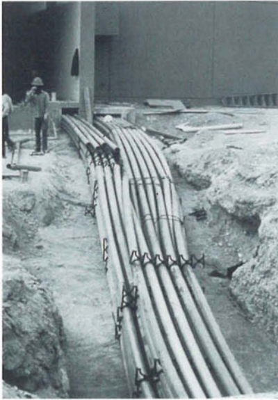
Utility ducts (left); a backfilled and compacted utility trench.
