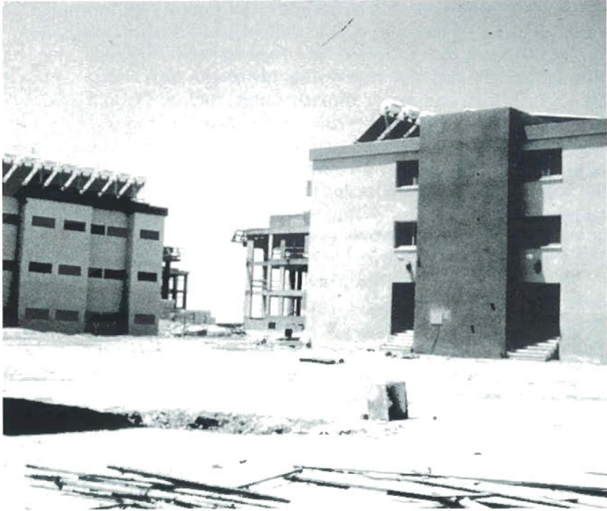
Airmen's dormitories, with solar panels on rooftops, at Ouda.
