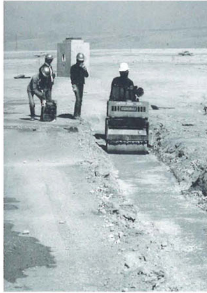
Utility ducts (left); a backfilled and compacted utility trench.
