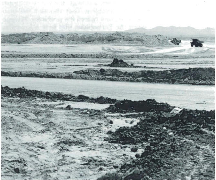
Excavation of Glide Path Hill at Ramon
