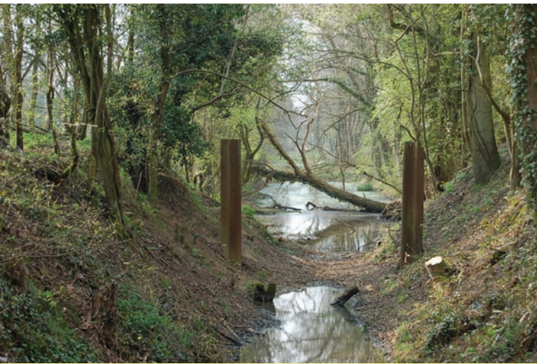
Southland Lock - the corner posts (quoins) are the only visible signs of the original lock
