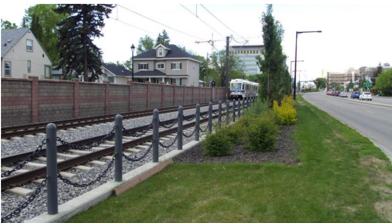
Figure 4.4.1 - LRT through Belgravia in Edmonton
