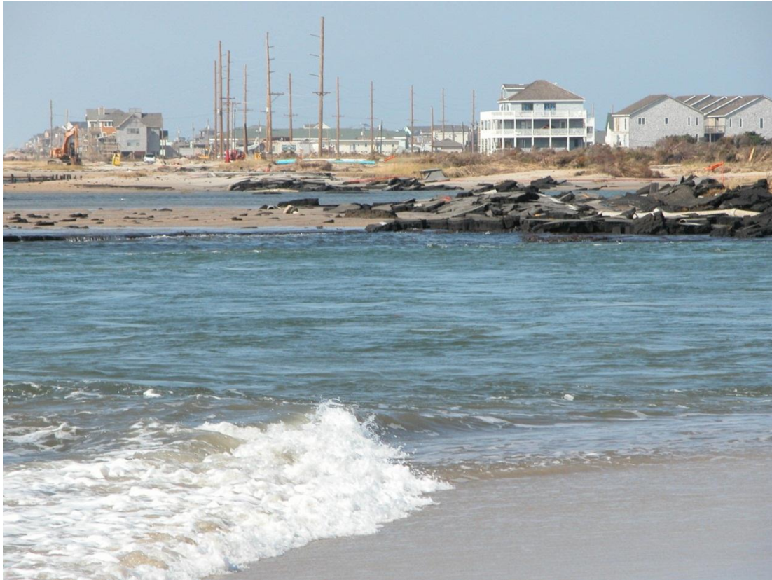
Figure 3. Storm surge, waves, and currents from Hurricane Isabel (August 2003) cut a breach across Highway 12, on Hatteras Island, North Carolina, severing the single road in and out of the village. The Atlantic Ocean is located to the left of the image. Asphalt from the highway is on the right side of the image. See figure 4 for aerial view of breach.
