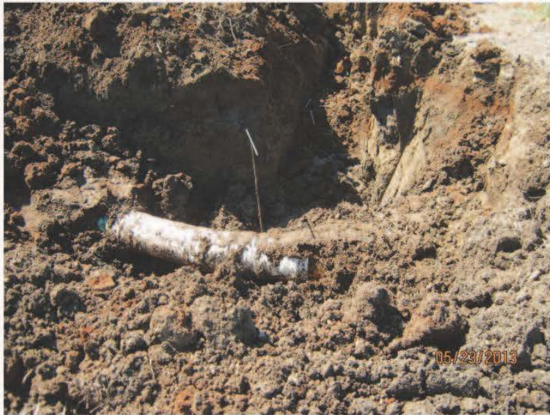
Step 1: Access Underground Line
