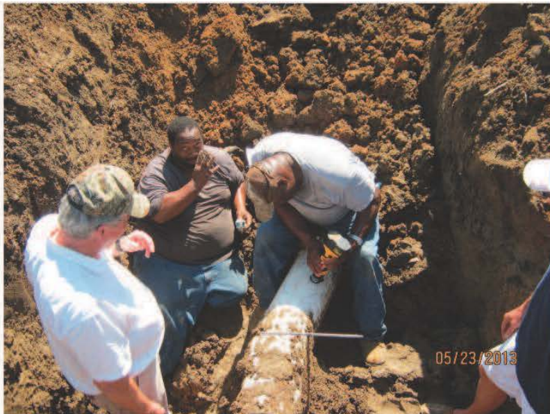
Step 2: Cut Appropriate Size Hole (See instalation specs)
