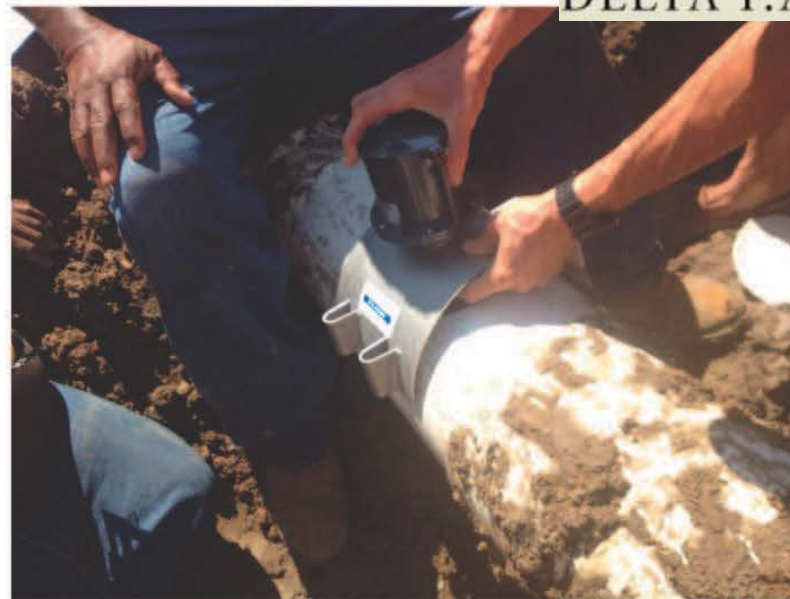
Step 4: Install Meter - continued
