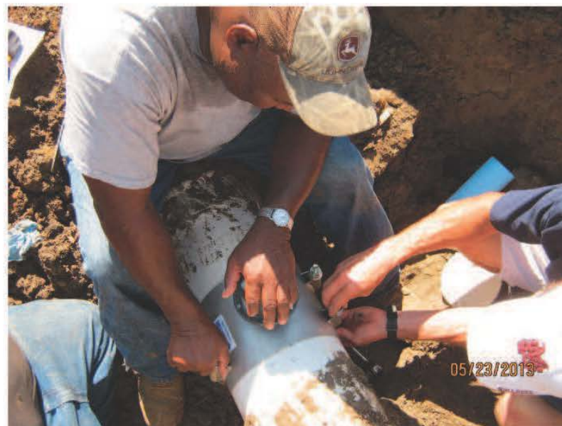
Step 4: Install Meter - continued
