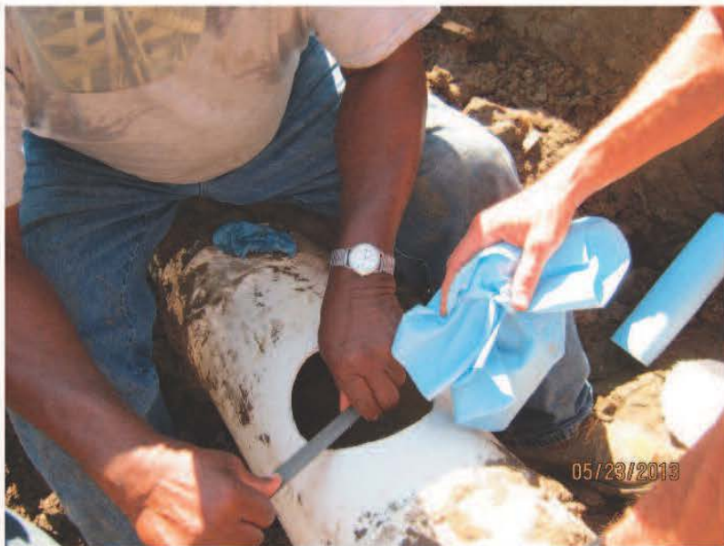
Step 3: Clean and check hole size
