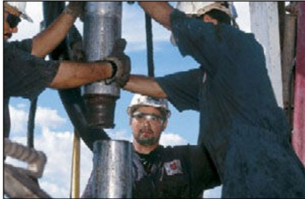
Installing Well Casing
