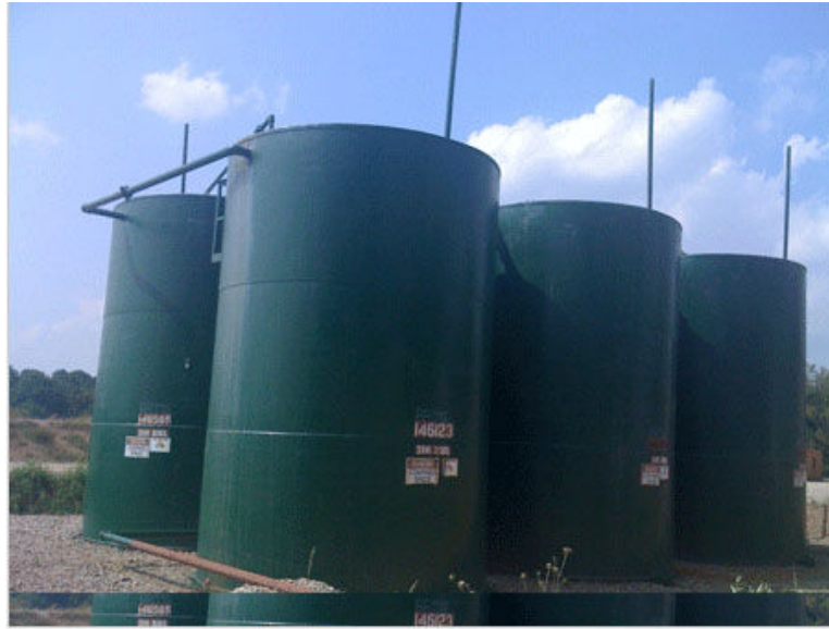
EQT Corp. brine water tanks (collect residual frac water as it returns to the surface over time) in Waynesburg, PA. Photo credit - Josephine Sabillon
