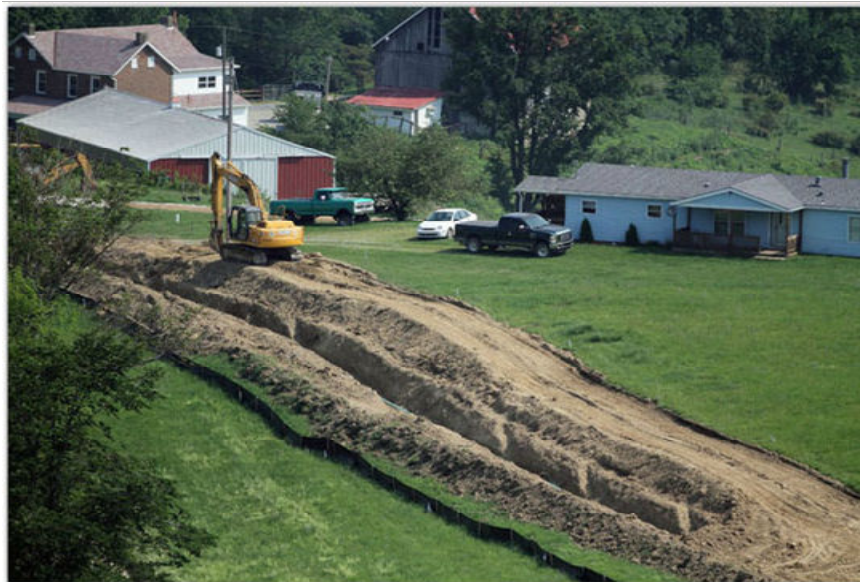
A pipeline laying operation near a home in Greene County. ( Michael Bryant / Staff Photographer )
